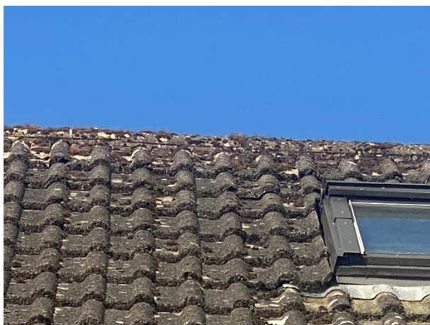
Building B10 PRF – Small cracks in roof tiles adjacent to skylight.
