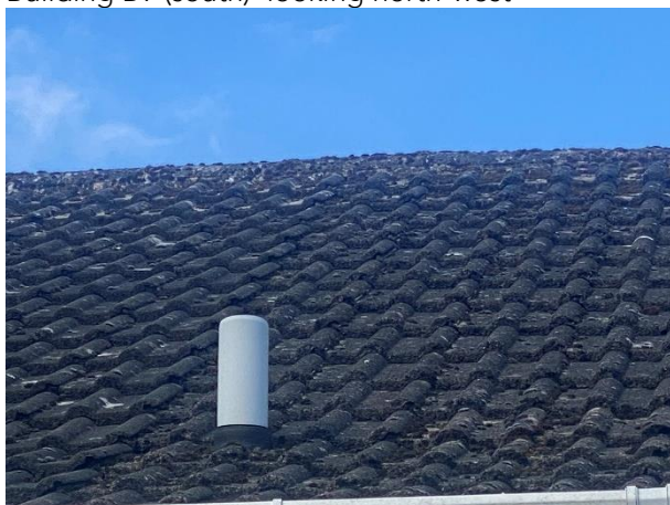
Building B10 PRF – Loose tiles along a ridge to the left of the ventilation pipe.
