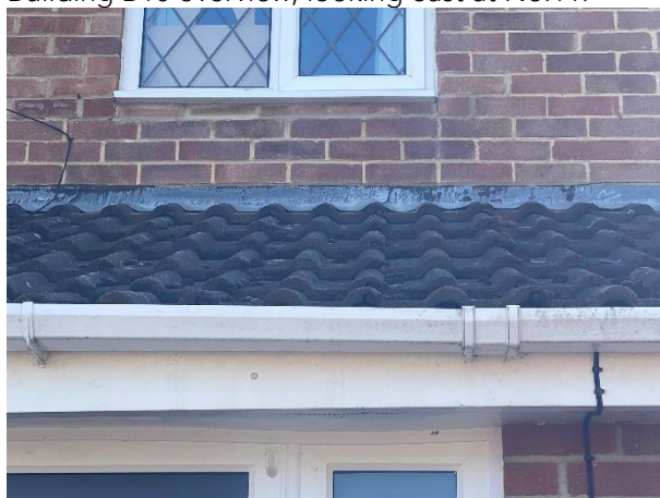
Building B10 PRF – western aspect raised roof tiles.
