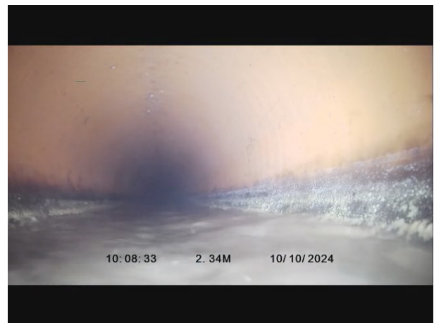
4, 00:00:14, 2.34 m Water level, 15% of the vertical dimension
