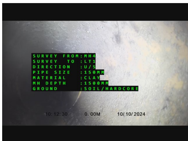
1, 00:00:00, 0.00 m Start node, manhole, reference: MH4
