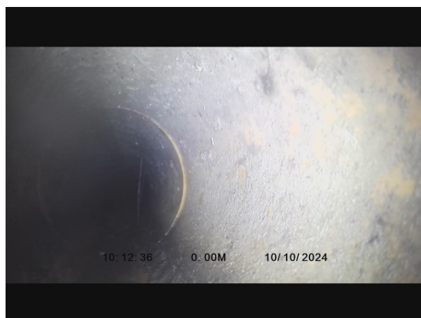
2, 00:00:06, 0.00 m Water level, 5% of the vertical dimension
