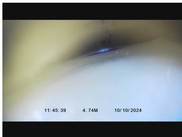
4, 00:00:44, 4.74 m Water level, 80% of the vertical dimension
