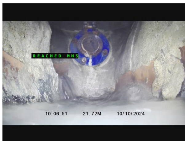
4, 00:01:13, 21.72 m Finish node, manhole, reference: MH5
