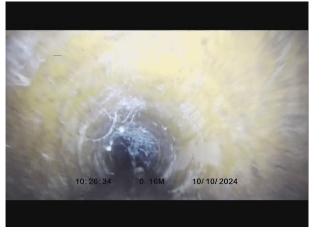
2, 00:00:04, 0.00 m Water level, 5% of the vertical dimension
