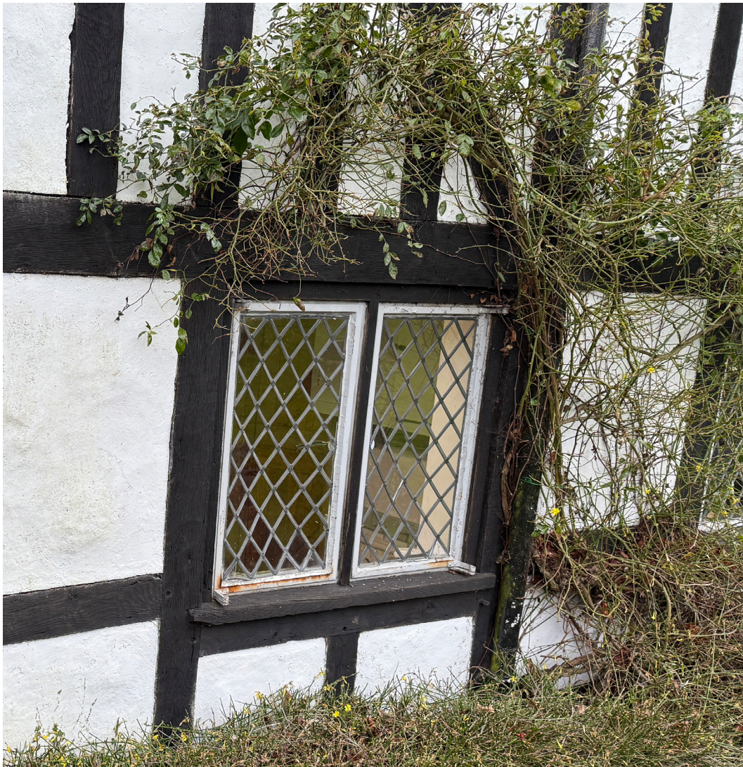
Existing window to be replaced
