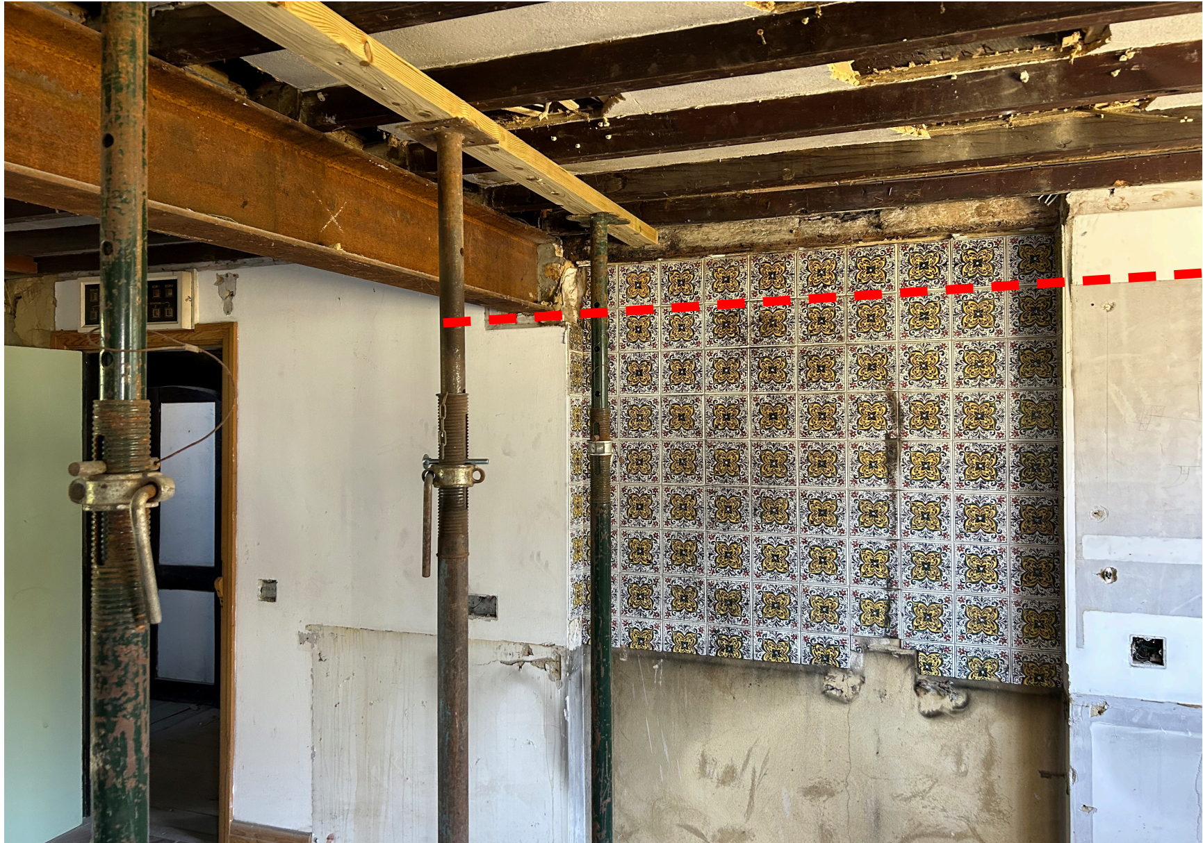
Fig. 9 - Photograph B: Spreader beam is not to impact 17th Century fabric, dashed line indicates spreader beam location.
