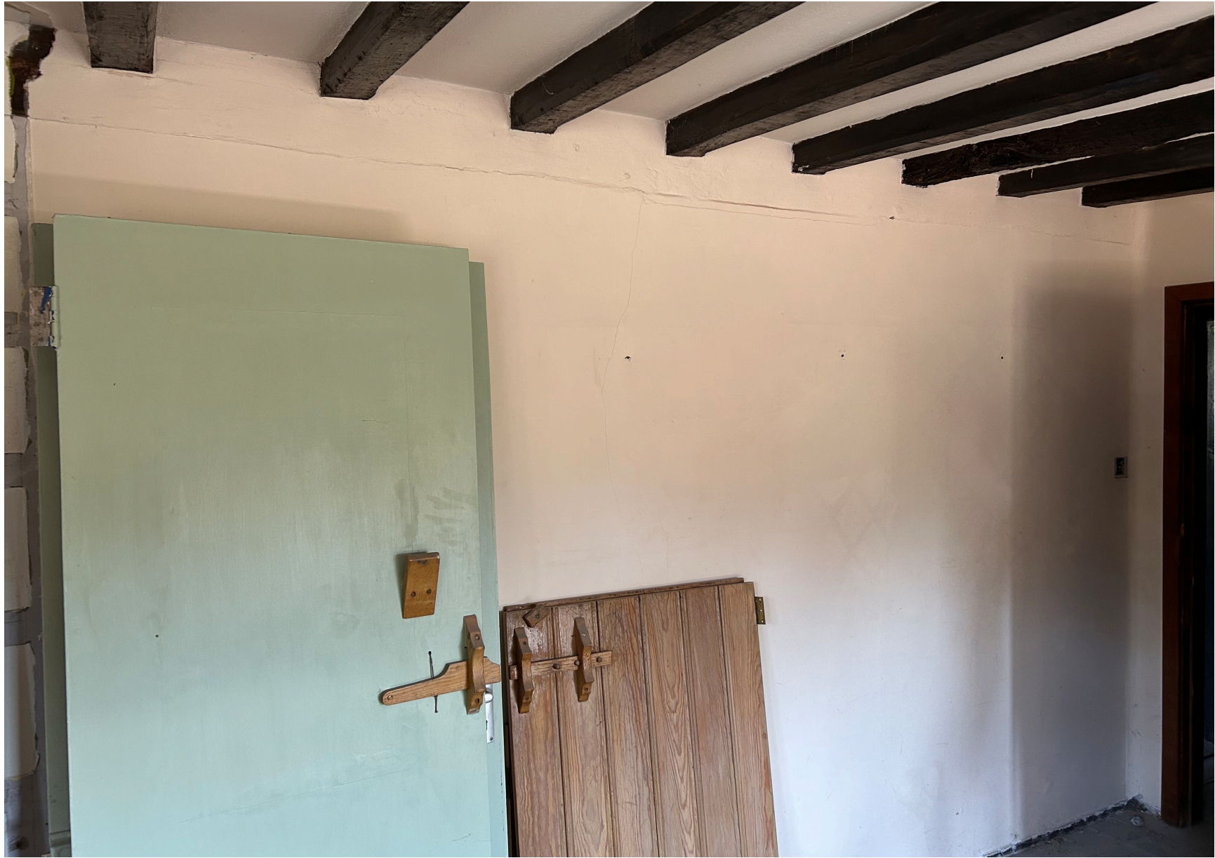
Fig. 8 - Photograph A: Showing existing wall and historic beam (likely 17th Century)
