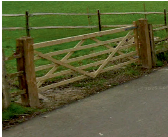
Five bar wooden gate, with pos and rail fencing and new hedgerow
