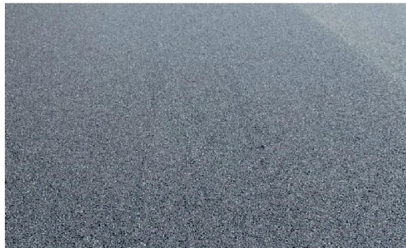
Tarmac for hardstanding
