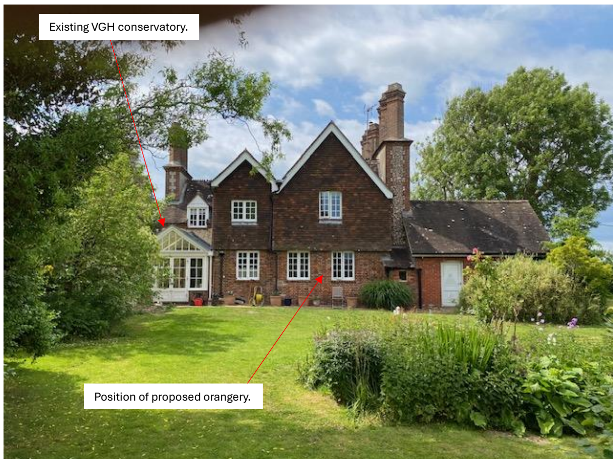
Fig. 8 – Photograph showing existing east facing rear elevation.
