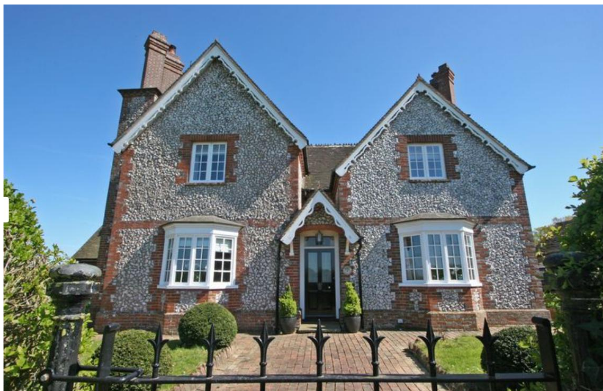
Fig. 1 - Bridgers Farmhouse principal elevation.
