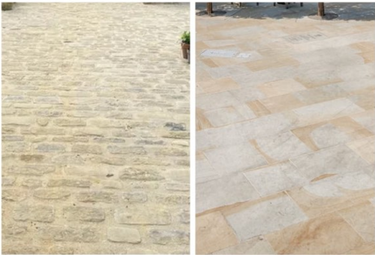
Left: Sawn Yorkstone paving slabs / cobbles creating a visual reference to historic existing sandstone flags.
