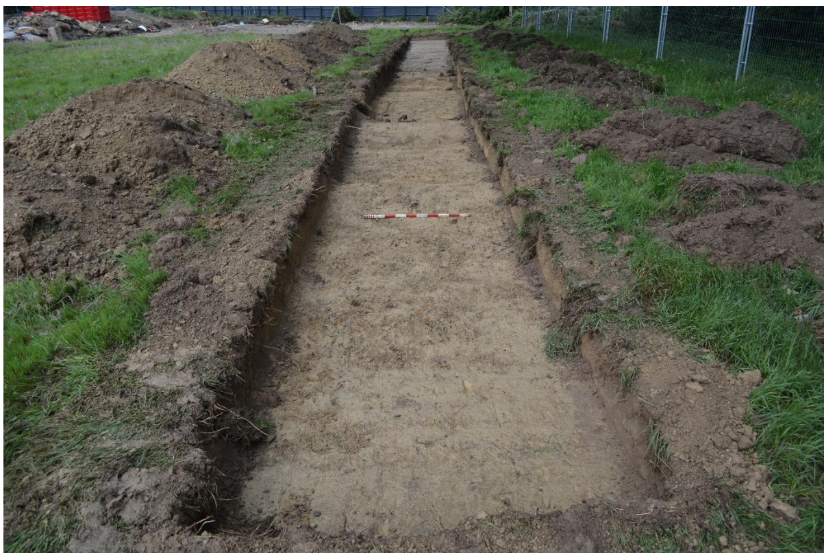
Plate 5. Trench 41, looking west. Scale 1m
