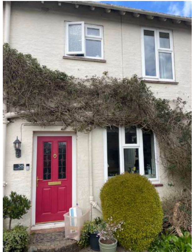
View looking west showing front elevation (partial)
