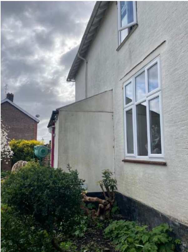
View looking east showing side elevation incl. lean to
