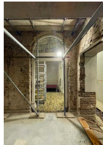
Opening to main stair hall
