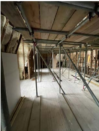
Looking towards east and north walls
