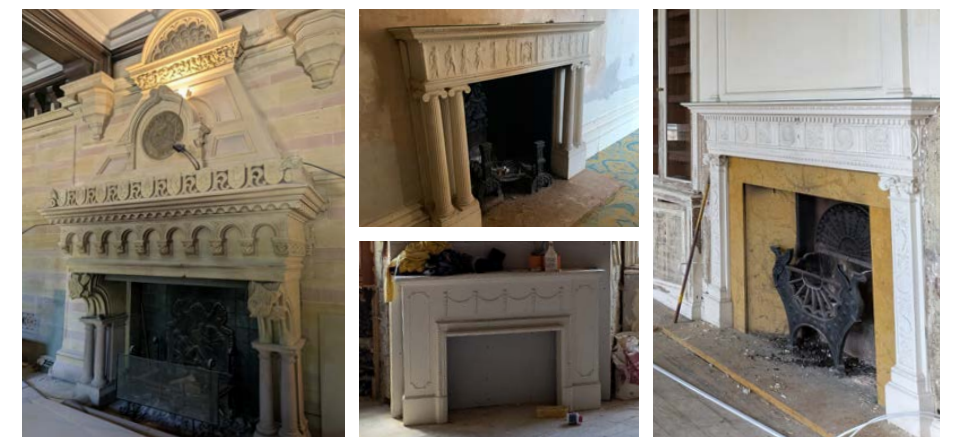
Fireplaces remaining in the property in other rooms
