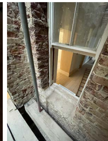
Window in west wall
