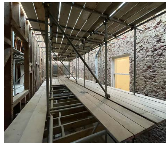
Looking towards east and south walls
