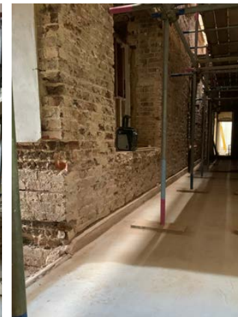
Lightwell south wall
