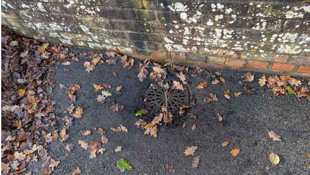
Existing sewer gully pot
