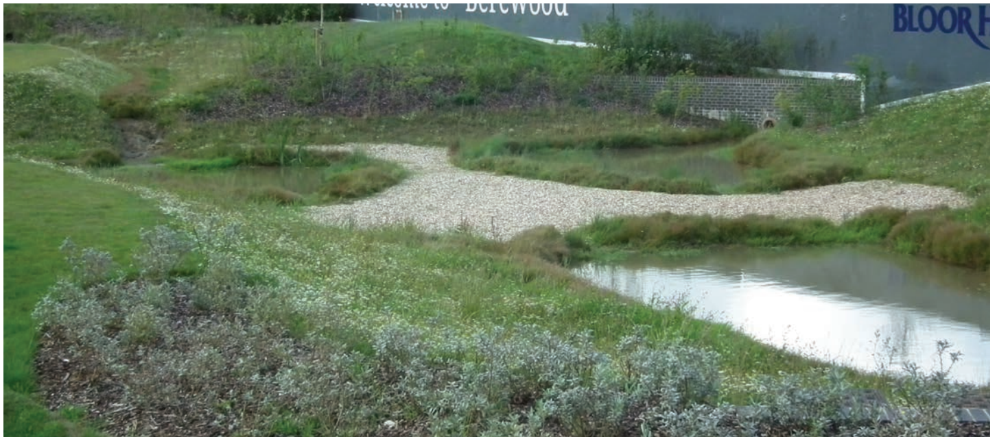
Vegetated pond under construction at Berewood
