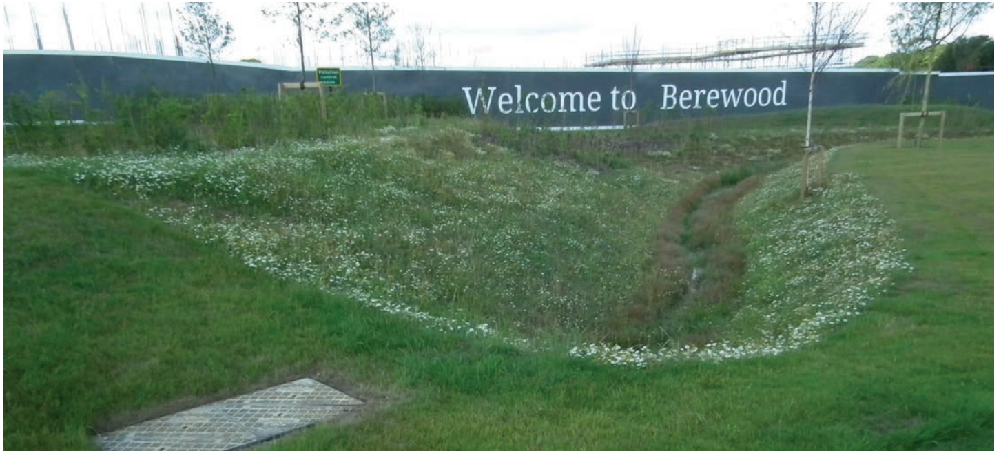
Swale under construction at Berewood
