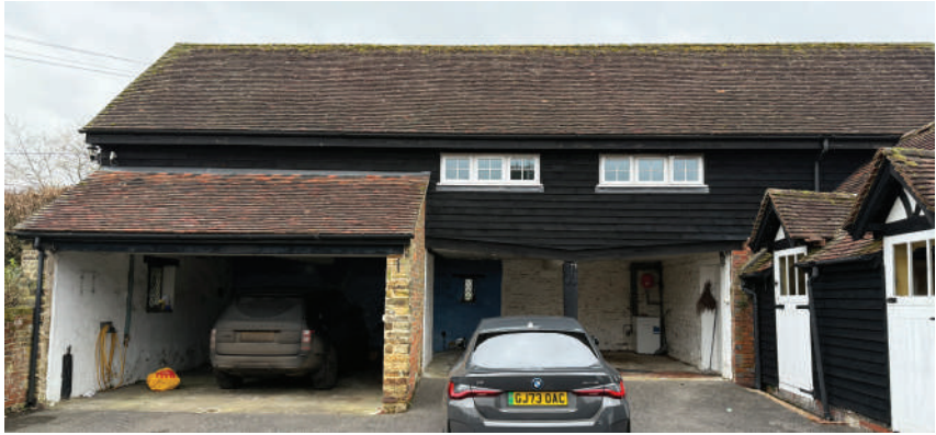
Existing eastern elevation to annexe & garage
