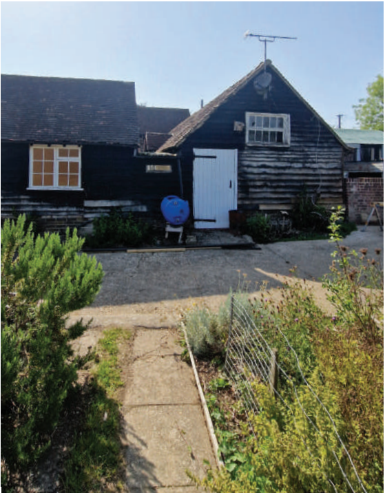
Eastern elevation (1950s extensions)
