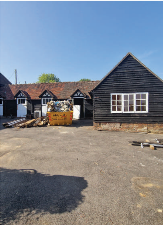
Southern elevation (C19th Stables & 1950s extensions seen)
