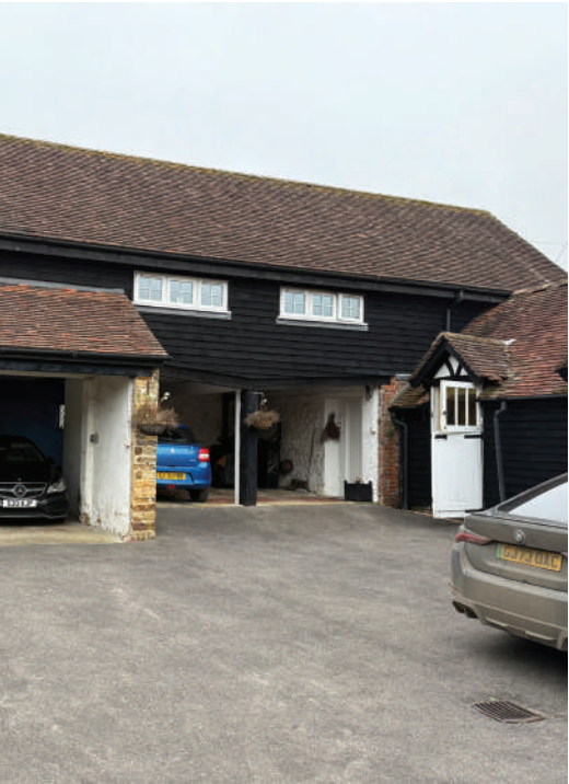
Former annexe (C21st above mid to late C17th Garage. 1950's lean-to extension to garage on left).
