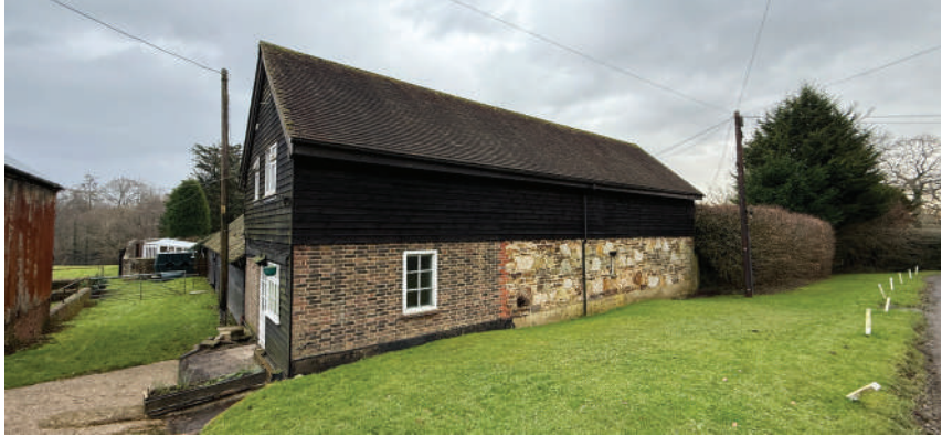
Existing western elevation: C17-18th Ashlar on right
