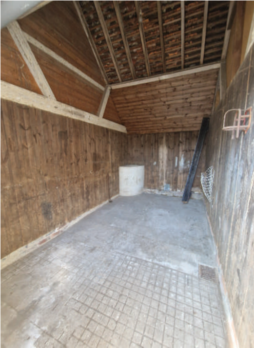
Existing stable bay with water trough shown in corner to be retained, as well as showing the roof trusses to be retained to denote the historic layout of the bays.
