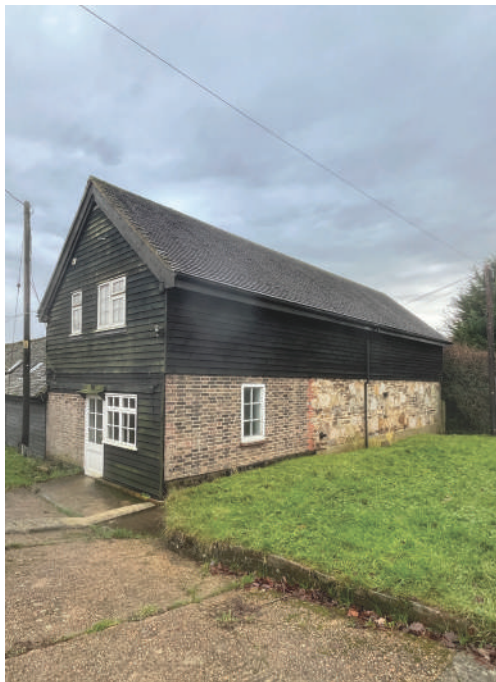
C17th-18th Ashlar wall below adjacent to contemporary additions/repairs to corner & 1F
