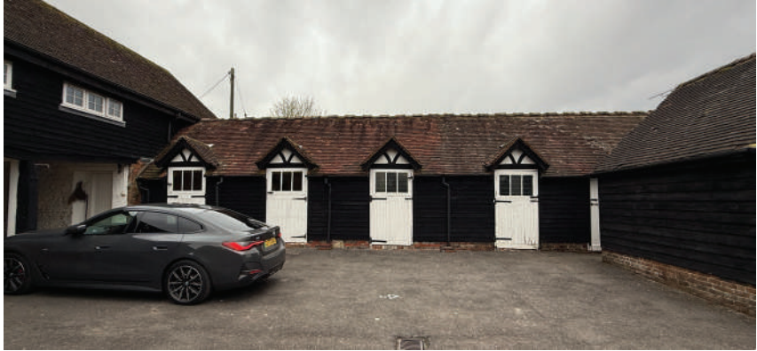
Existing south facing elevation to stable bays
