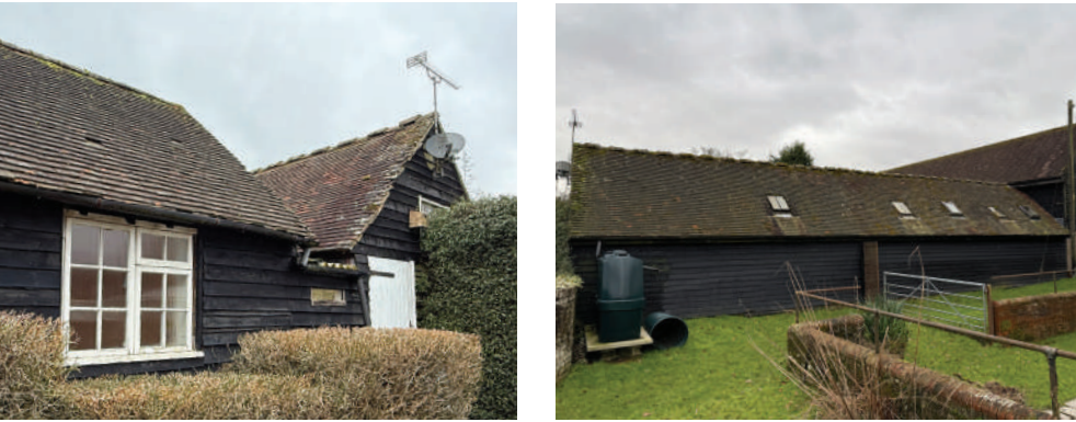
Examples of existing roof tile condition
