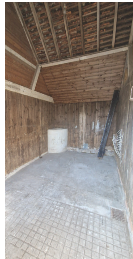
Example of one late C19th stable bays with cement water trough of low significance across each value
