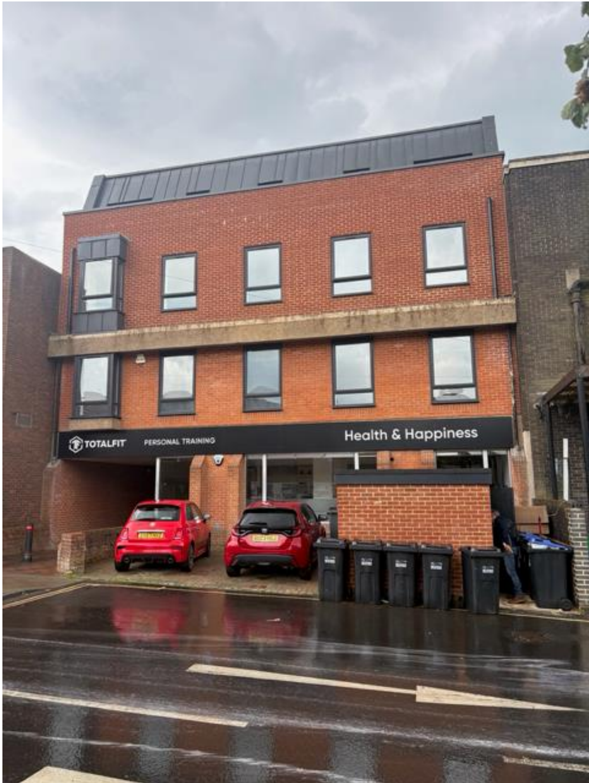
Building North Elevation, showing brick built cycle store
