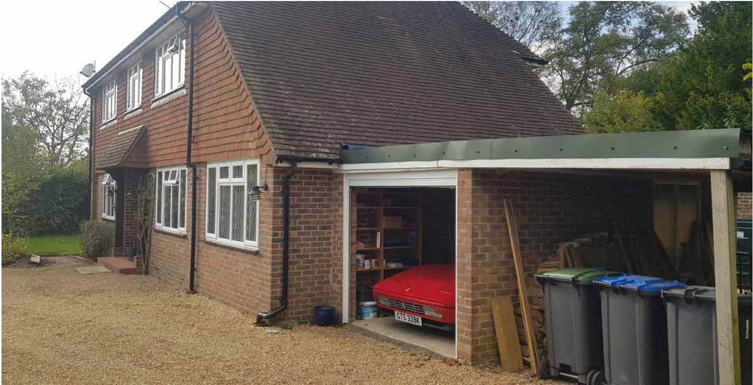
Photo showing existing garage and carport (prior to addition of approved porch)
