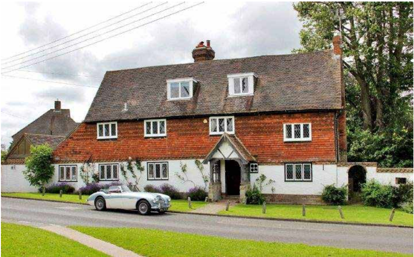
Rixons, Grade II Listed Building (with view of Mulberries Roof beyond)
