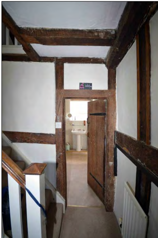
Plate 11: The in situ and unaltered doorway in the T2 truss on the first floor
