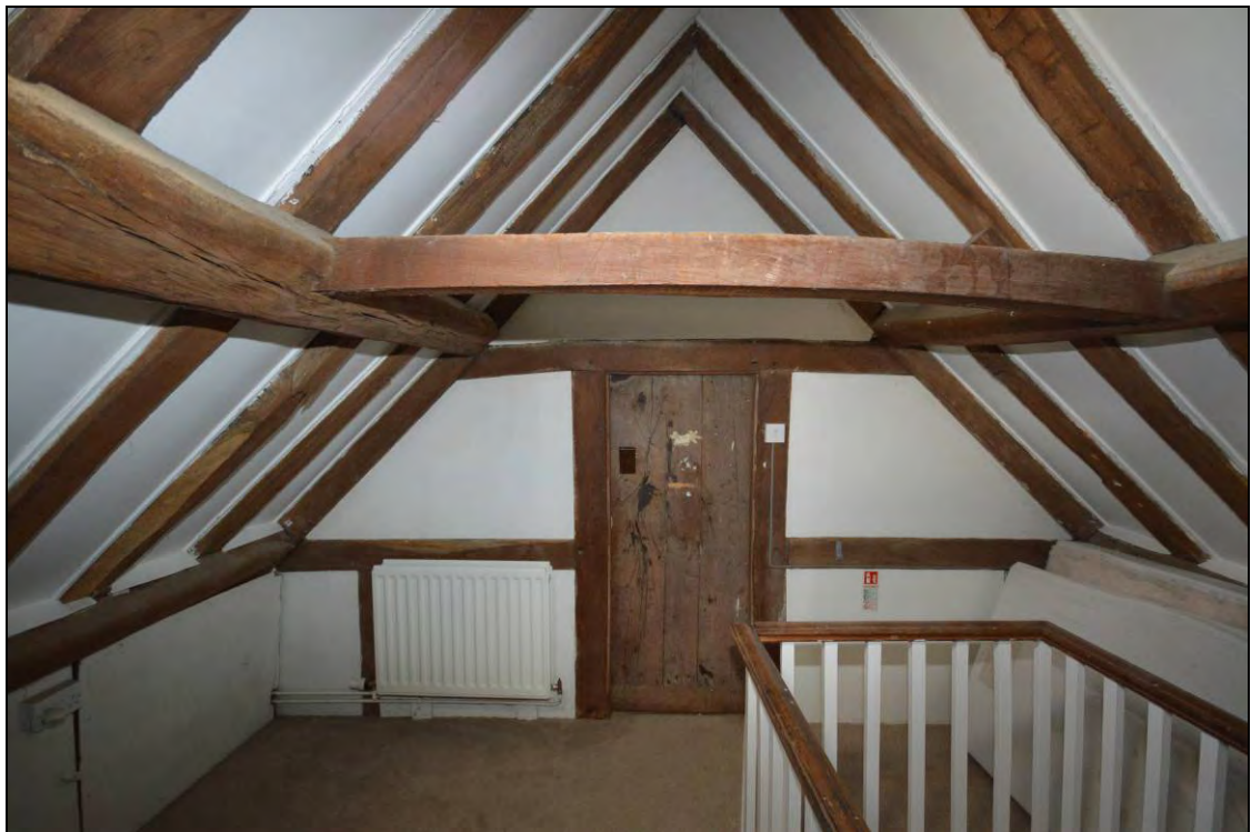
Plate 20: The T2 partition truss of queen stud type
