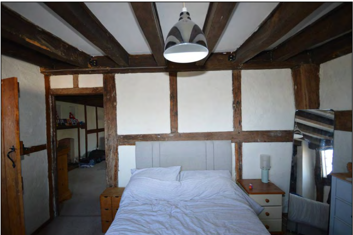
Plate 3: Small panel framing in the T4 truss between bays 3 and 4 on the first floor
