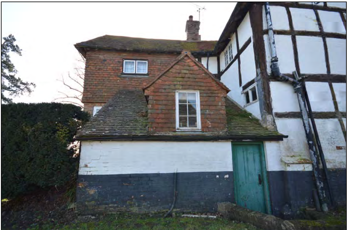
Plate 26: The current structure at the junction of the main range and rear wing at the north end of the house: the doorway provides access to the cellars, the dormer window lights a ground floor room, illustrating the sloping topography of the site
