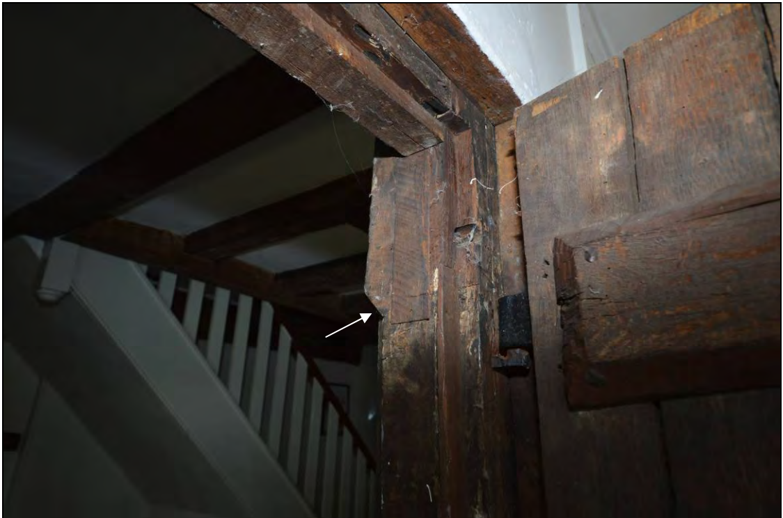
Plate 10: The mortise and tenon for the door-head of the ground floor doorway in the T2 truss, note also the mitred corner still visible at the top of the chamfer, indicating the level of the soffit of the door-head (arrow)
