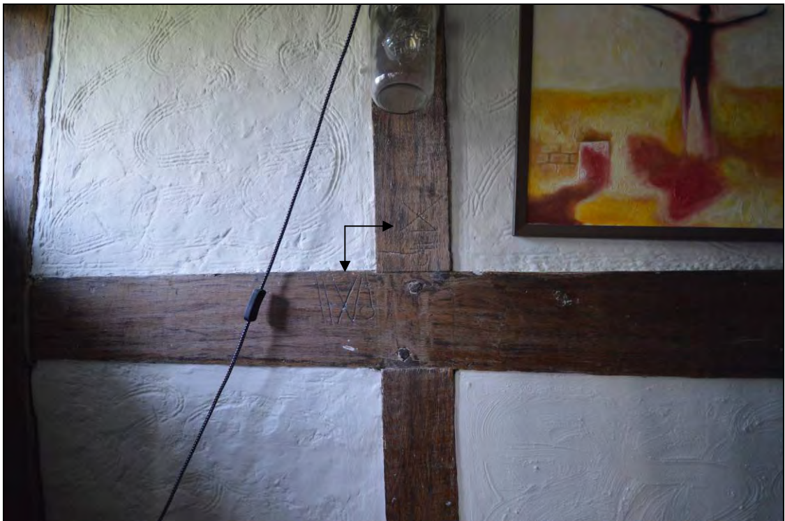
Plate 5: Comb-decorated daub with lime-skin on the south side of the T4 truss facing into the hall chamber in bay 3. Note also the carpenter's marks at the junction of the rail and studs (arrow)
