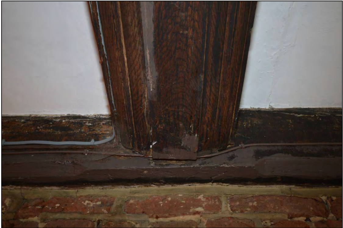
Plate 13: Double ovolo-mouldings to the girder in the ceiling over the parlour in bay 1
