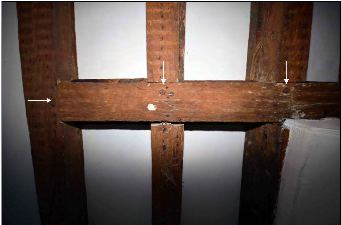
Plate 18: Detail of the original in situ trimmer for the staircase in bay 4, between ground and first floors, all original members are jointed and pegged in place (pegs indicated by arrows)
