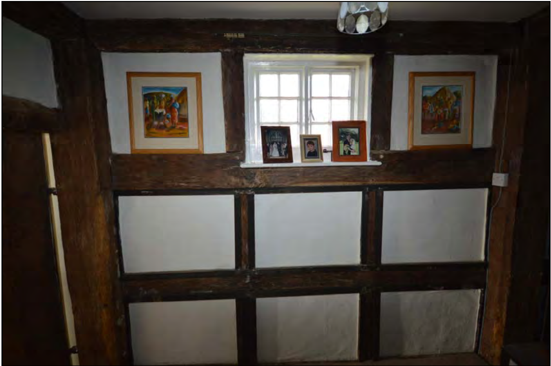
Plate 38: Metal strapping on the frame to the west side of bay 2, first floor
