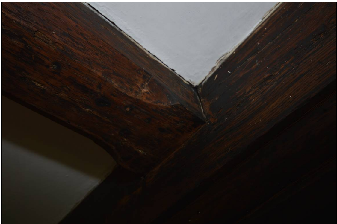
Plate 14: Step-and-hollow chamfer stop to the bays 1 and 3 joists (ground floor)
