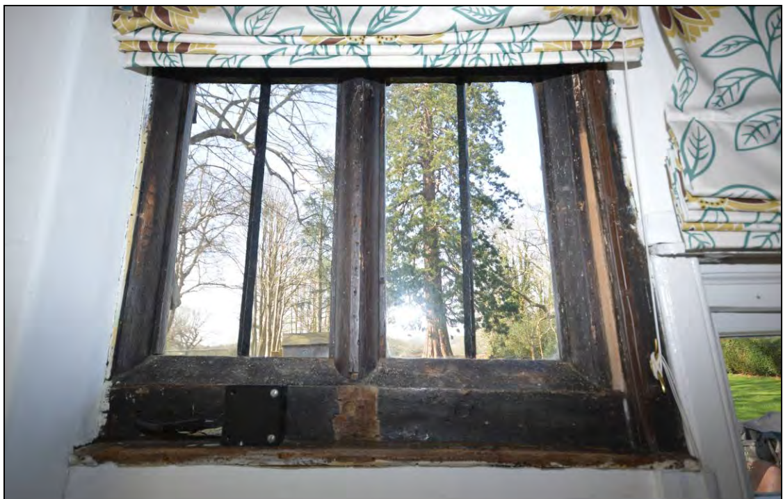
Plate 8: Detail of one of the two-light ovolo-moulded windows
