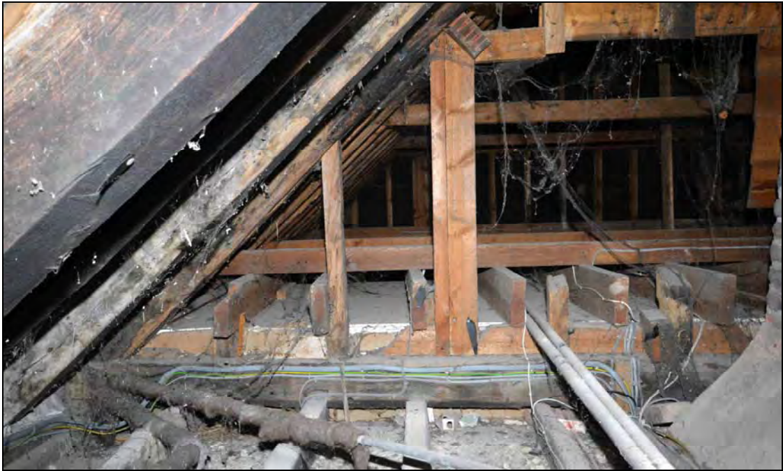
Plate 24: View into the rebuilt roof at the eastern end of the rear wing
