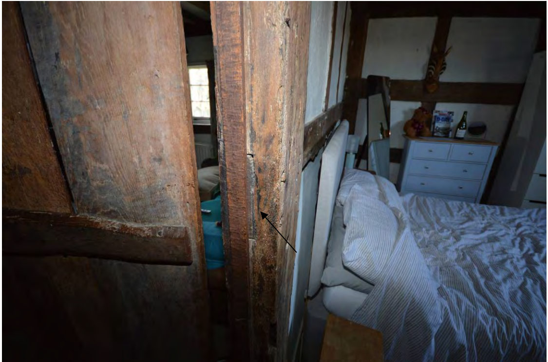
Plate 9: The mortise and tenon for the continuation of the rail (arrow), exposed when the rail was removed to create a doorway between the bay 3 and 4 first floor rooms
