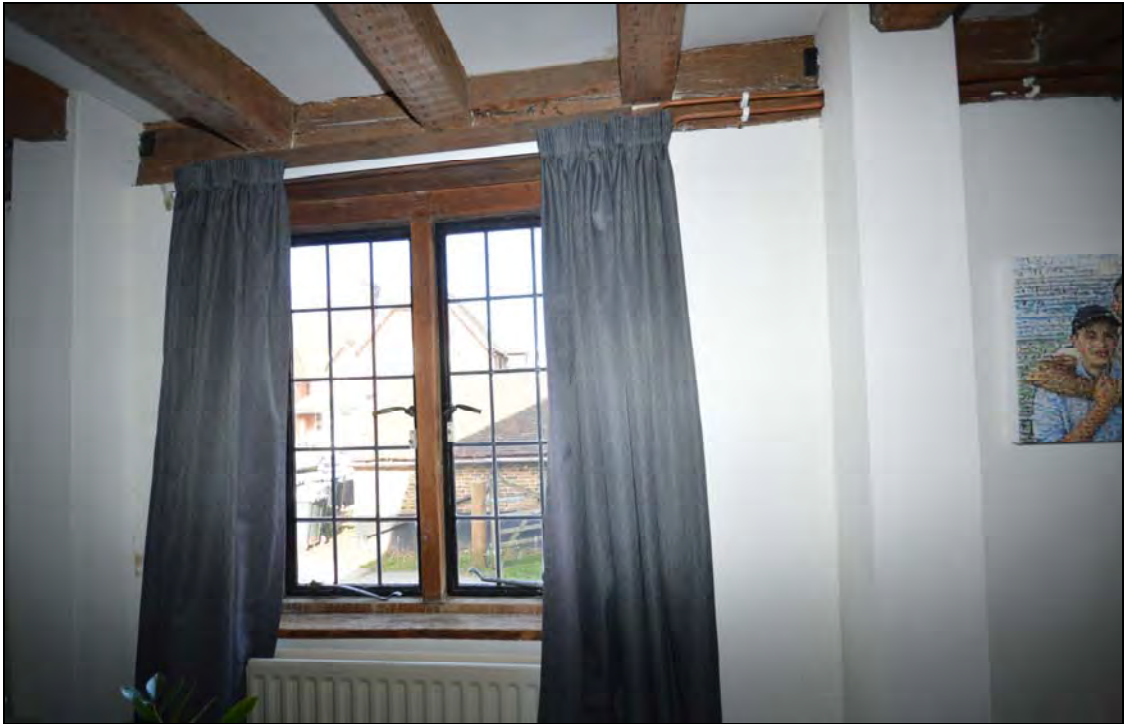
Plate 36: Intervention to strengthen the south end of the main range, ground floor
