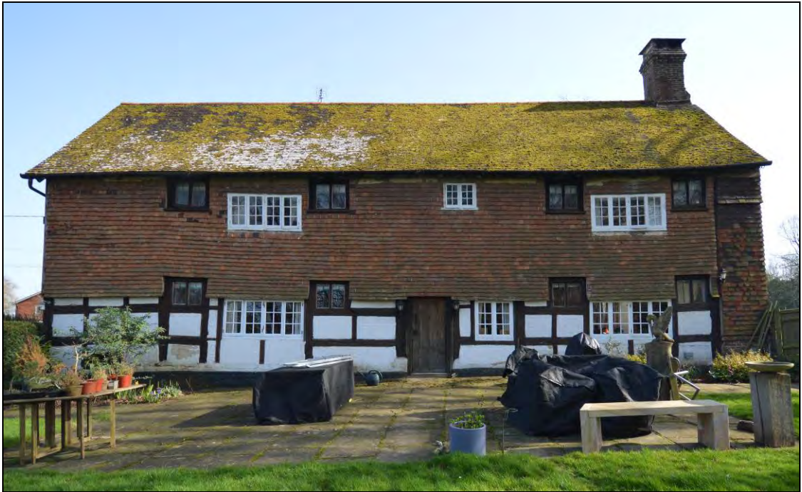
Plate 7: Eight surviving ovolo-moulded-mullioned windows on the west elevation of the main range
