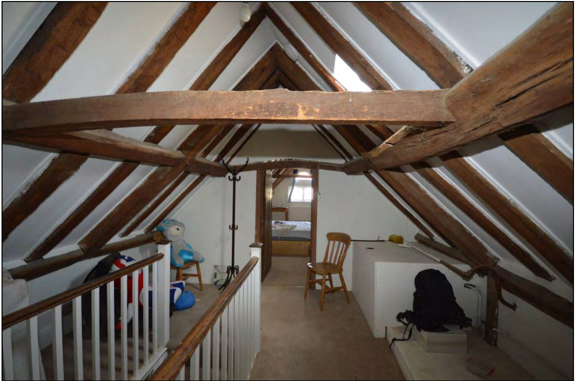
Plate 19: Two tiers of butted side purlins in the main range roof
