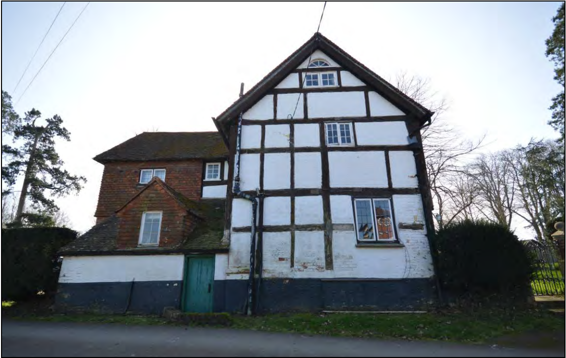
Plate 2: Small panel framing to the north end of the house
