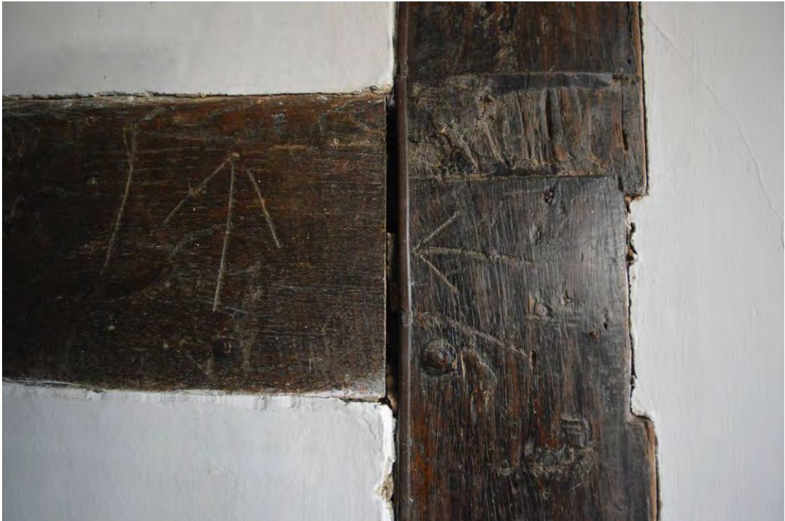
Plate 4: Example of the carpenter's marks on the T3 truss facing north into bay 3
