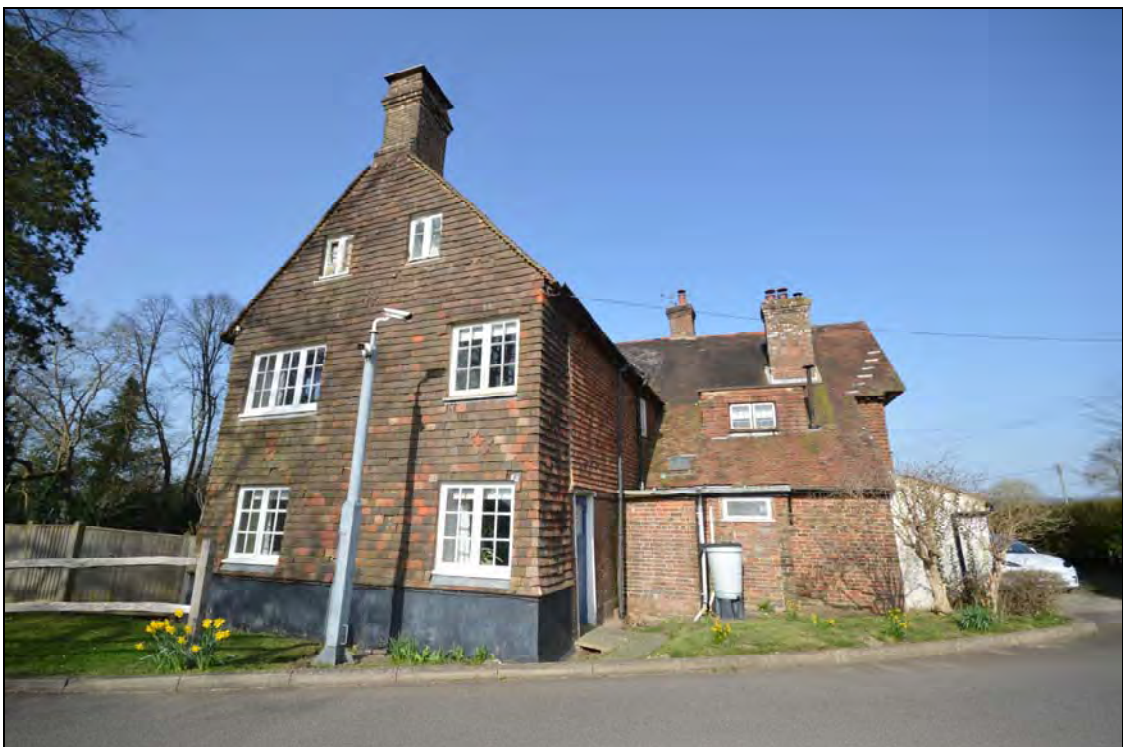
Plate 22: The south end and part of the east elevation of the main range showing the tile-hanging
