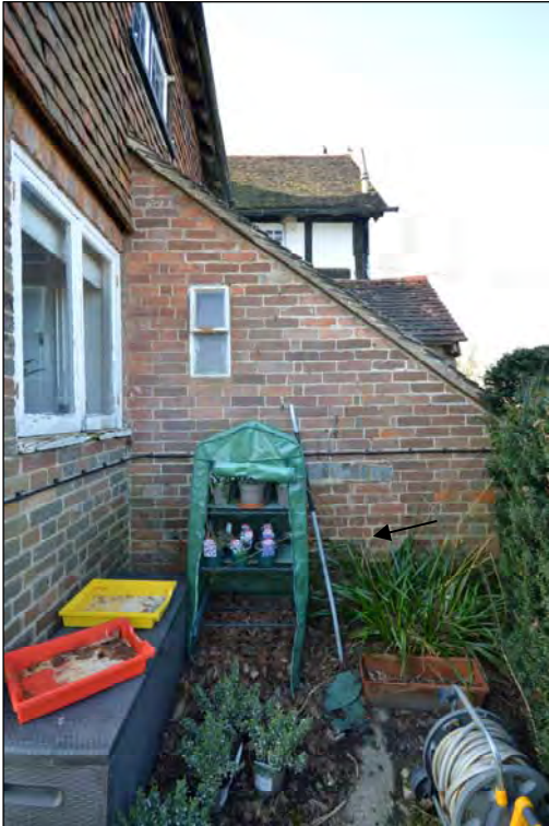
Plate 27: The east end of the group, in stretcher bond brickwork with the blocked cellar window at the base indicated by the over-fired headers of its arch (arrow)
