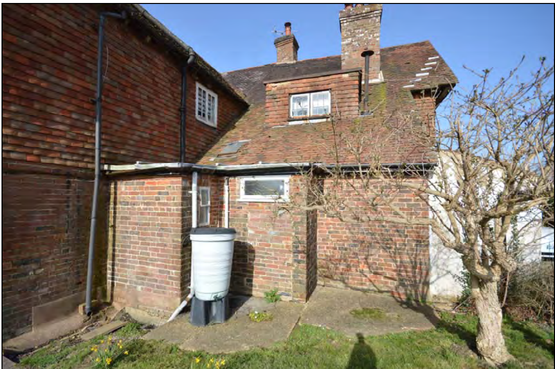
Plate 28: The south extensions with their flat-roofs, added to the group after 1968, in addition to the flat-roofed dormer inserted into the earlier lean-to that abuts the rebuilt rear wing
