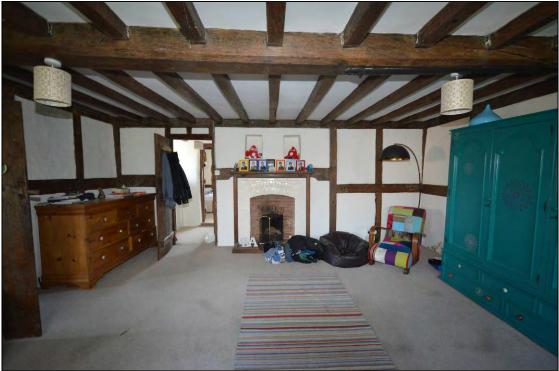
Plate 16: The bay 3 first floor fireplace, with glazed brick insert surmounted by the bressumer of the original opening
