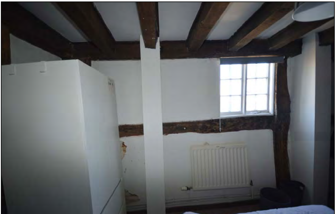
Plate 37: The continuation of the inserted supports at the south end of the main range on the first floor
