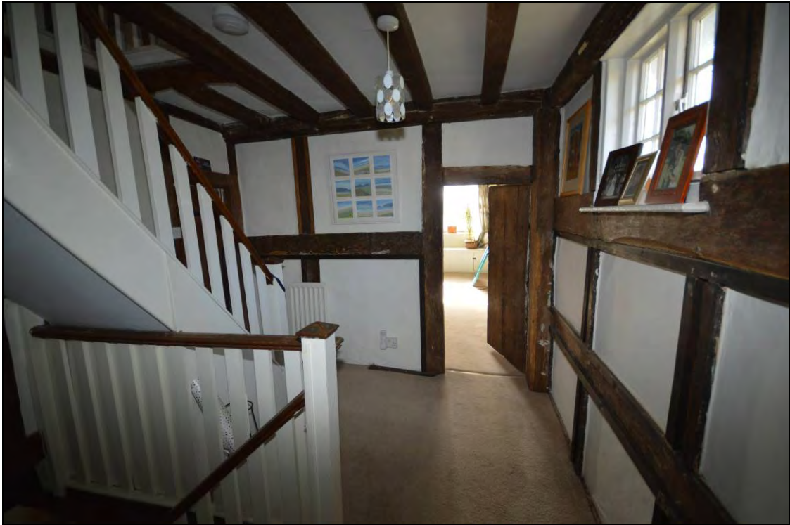
Plate 11: The in situ and unaltered doorway in the T2 truss on the first floor
