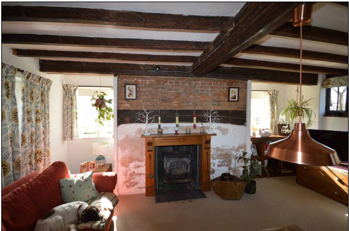
Plate 15: The ground floor fireplace in bay 1 with the bressumer of a much larger fireplace above the later insertion
