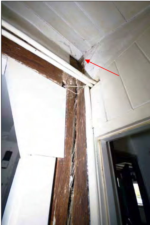
Plate 1: Detail of the L-shaped post at the junction of the main range and its integral cross-wing (arrow)
