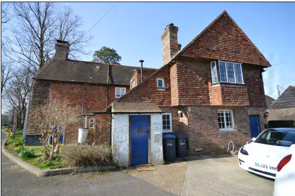
Plate 25: The rebuilt eastern end of the rear wing and the extensions added to it
