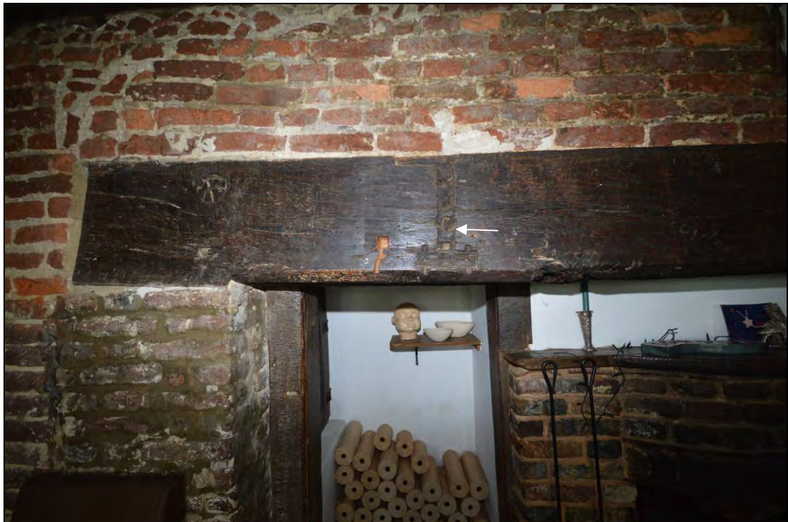
Plate 17: Detail of the bressumer over the bay 3 ground floor fireplace showing the scar made by the removal of the clock jack (arrow)
