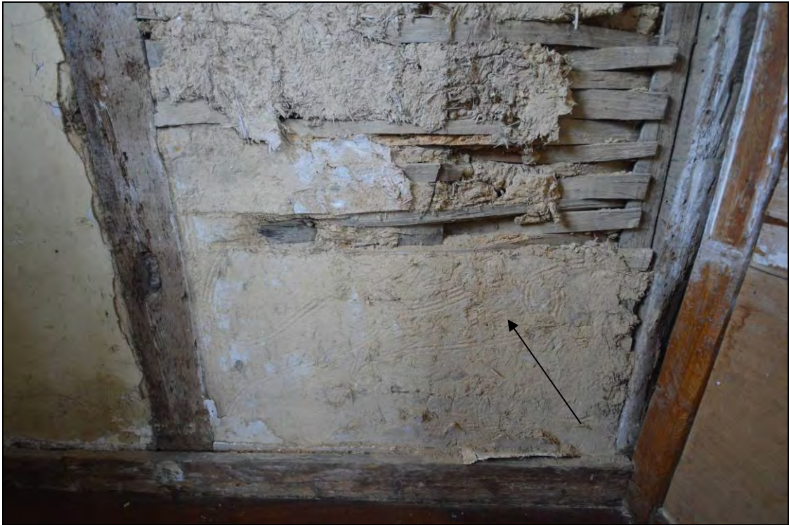
Plate 6: Lath and daub within the panels of the T4 truss (now within a bathroom) showing the remains of the comb-decorated daub (arrow)
