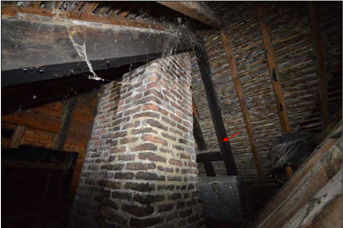
Plate 23: The chimney bay at the junction of the main range and its rear wing showing the remains of the original roof structure, rafter pairs and a butted-side-purlin on the south slope of the roof (arrow)
