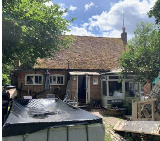
Existing Rear facade
