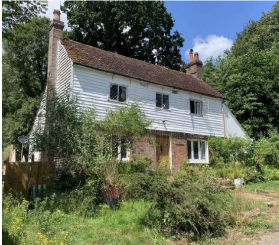
Existing Front facade
