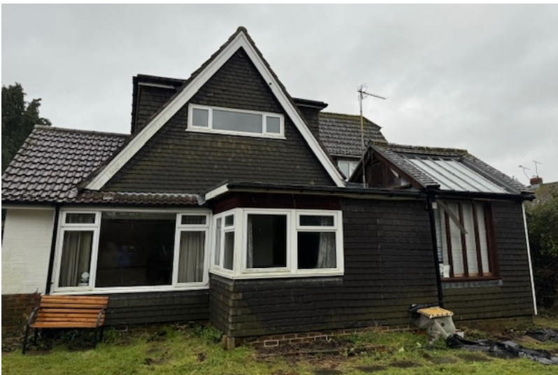
View of the house from the rear.
