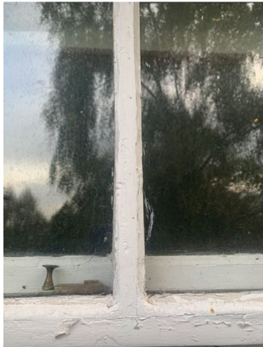
These are the oldest windows are are mainly held together with filler. They have been renovated over the years, but it is not possible to repair them further. They are never opened as they are so fragile
