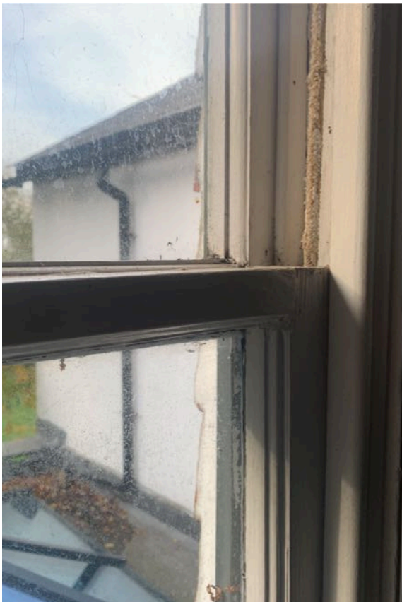
WINDOWS C1 - C3: Single glazed central bar sash windows with secondary glazing
