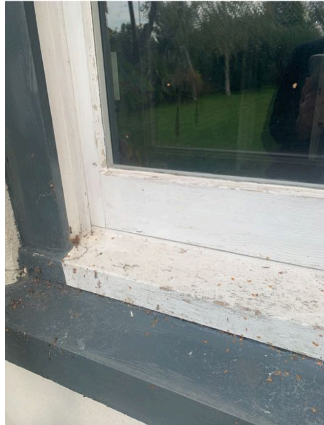
WINDOWS E1 - E9: New single glazed centre bar sash windows. These are renovated almost yearly, but because they are such poor quality soft wood, the paint is constantly cracking and they need regular maintenance.
