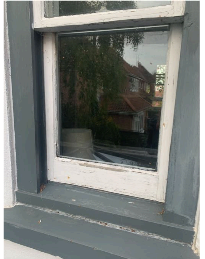
WINDOWS E1 - E9: New single glazed centre bar sash windows. These are renovated almost yearly, but because they are such poor quality soft wood, the paint is constantly cracking and they need regular maintenance.
