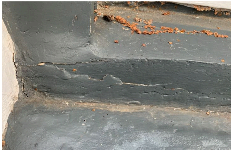
These are the oldest windows are are mainly held together with filler. They have been renovated over the years, but it is not possible to repair them further. They are never opened as they are so fragile
