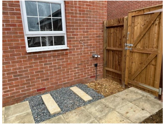
Picture: showing a plot ready for an ASHP installation.
