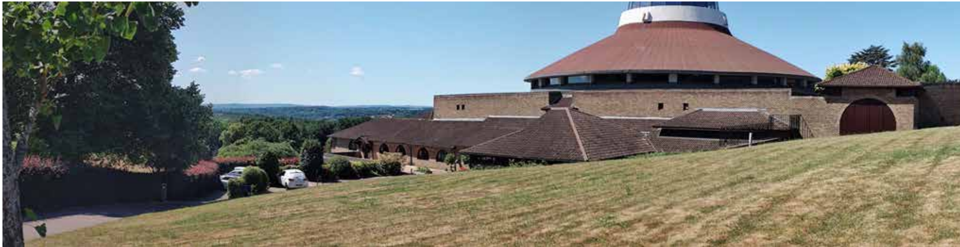
Photograph A - View of Worth Abbey from the south-eastern extent of the Site, looking south-west, demonstrating a localised open character with views of the High Weald National Landscape.
