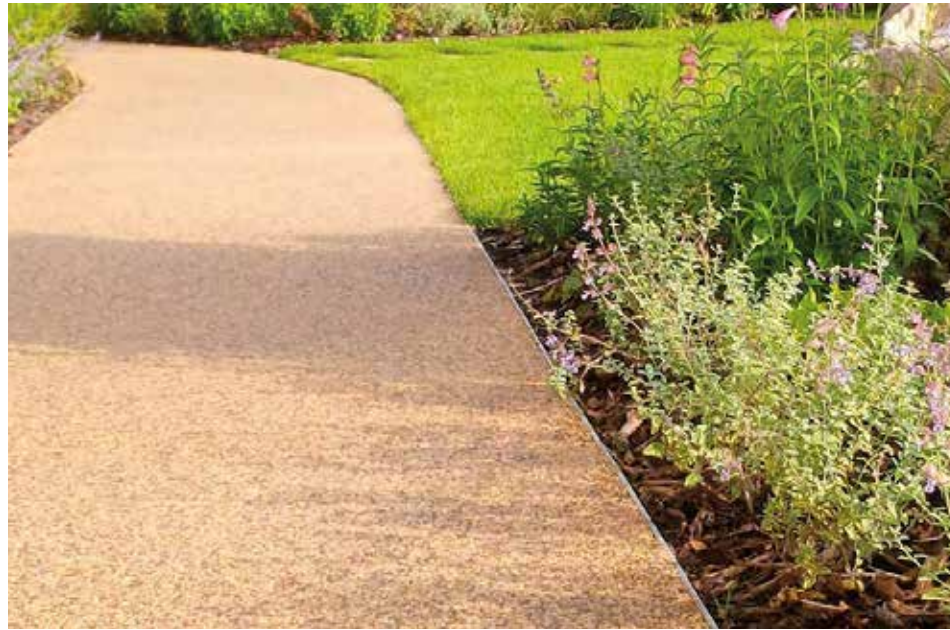
Pathing Surface Treatment: Aztec Gold - Resin Bound Gravel by; Retained by: Aluminum Edging.
