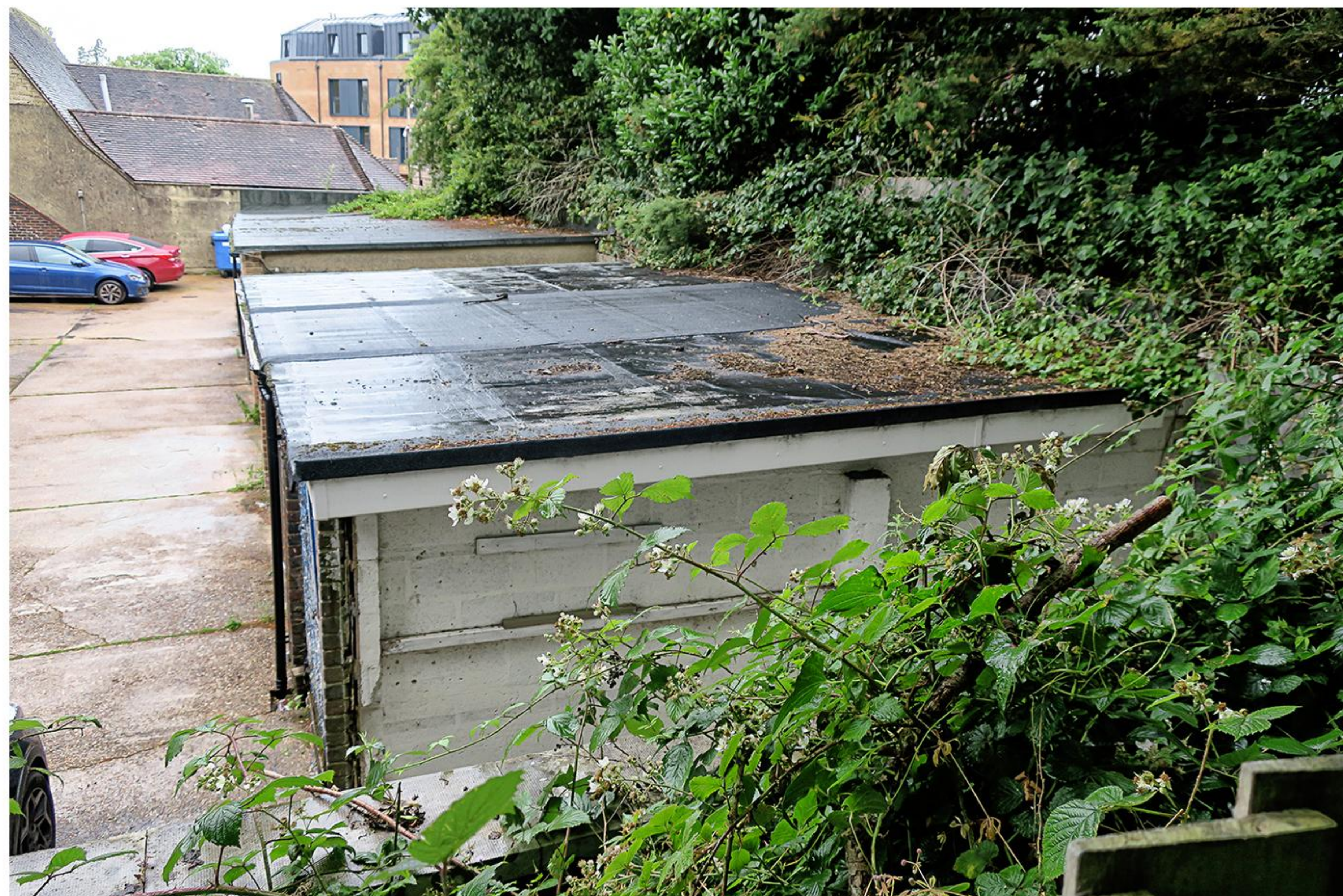
View from footpath looking West
