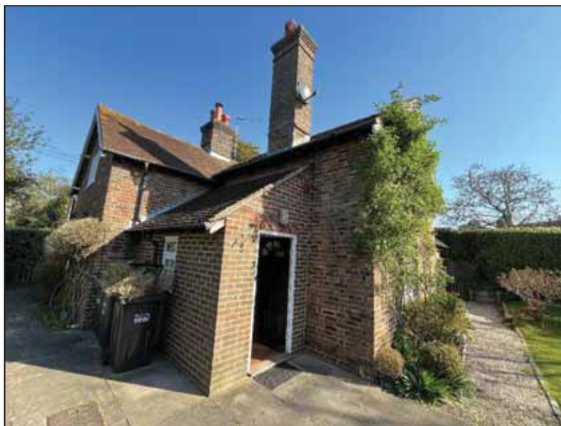
Image 12: Modern lean-to extension
