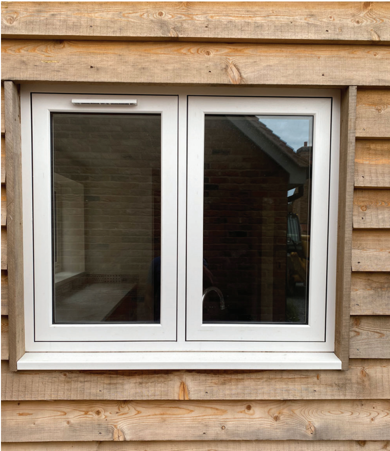
New Timber Windows
