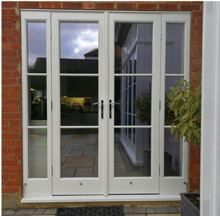
New Timber Windows
