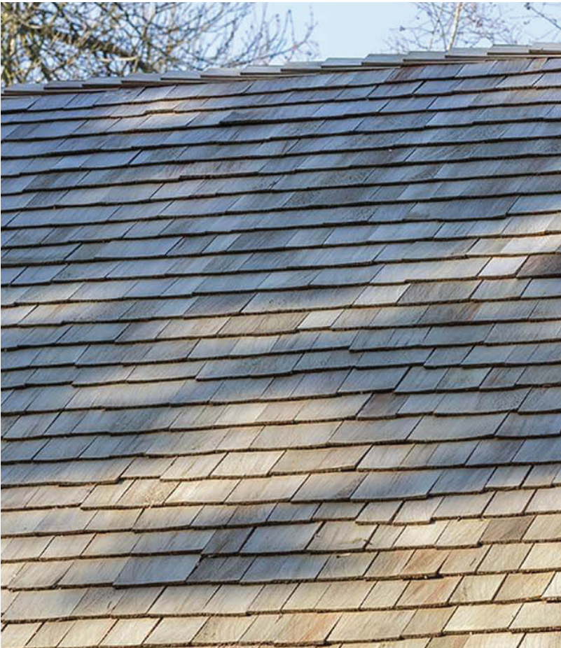
New Timber Single Roof
