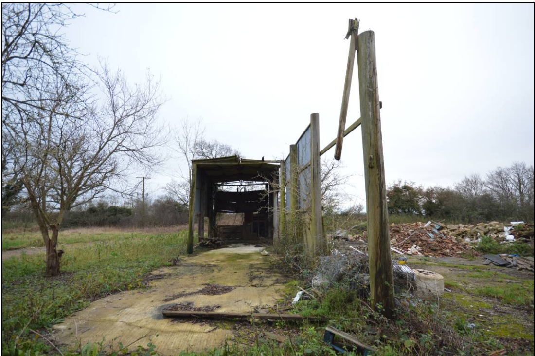
Plate 15: Barn 4, looking east, showing the poles at regular intervals that had supported the cladding and roof structure
