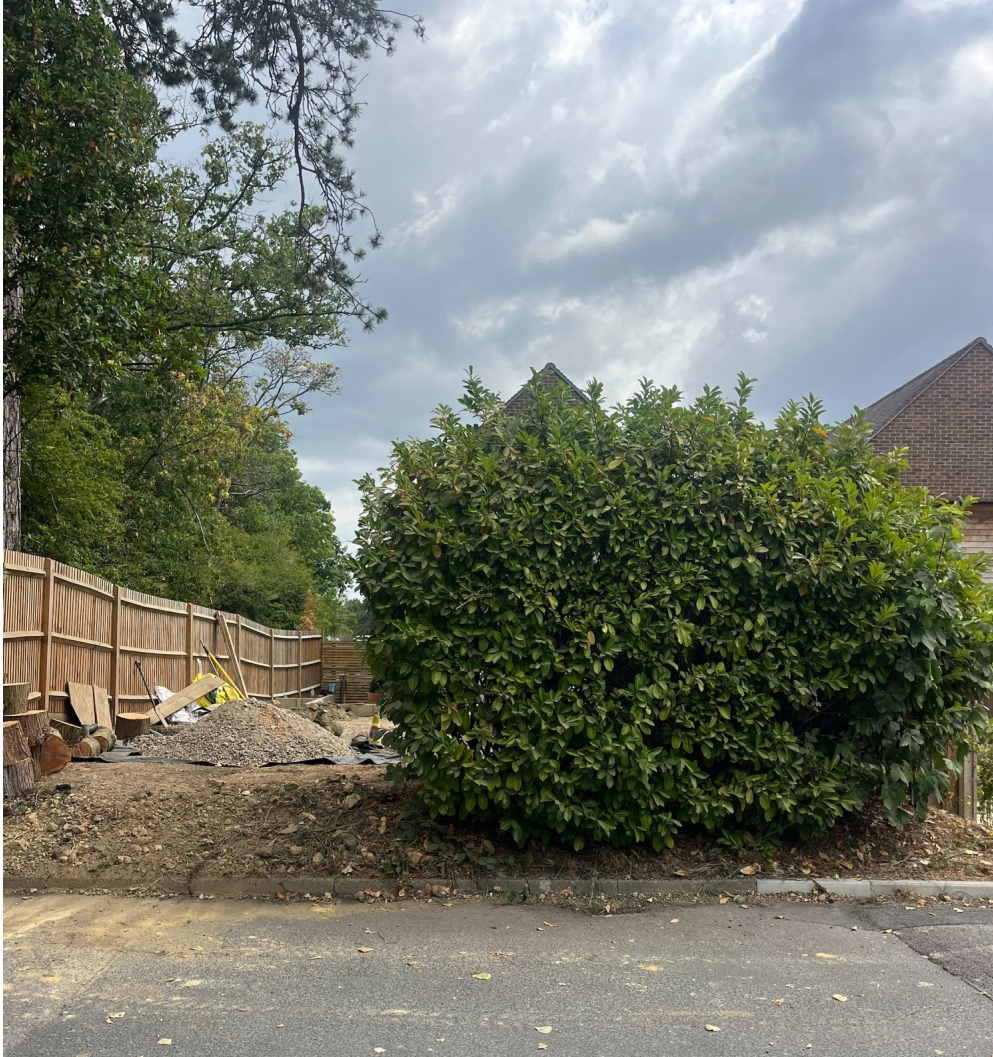
Figure 2.2 – Photo from footway on access road, showing location of pergola obscured by existing hedge on access road verge (n.b. fence temporarily removed to allow tree removal works)
