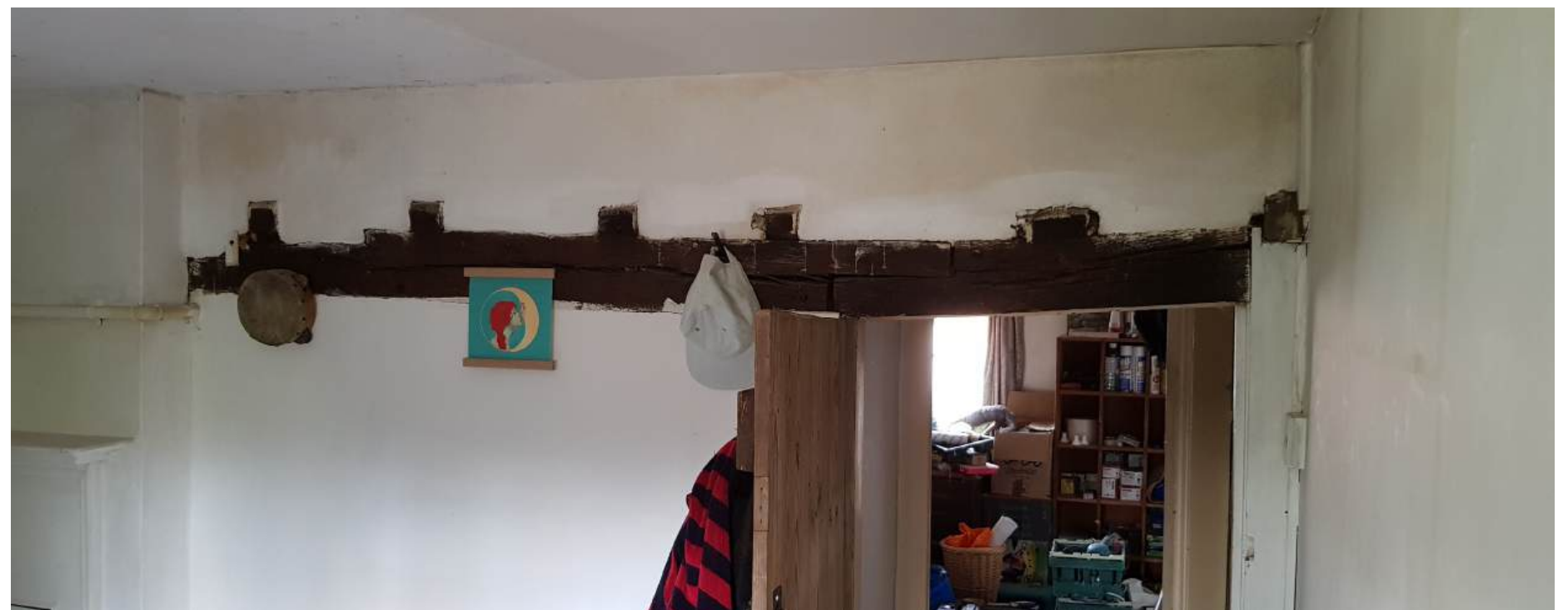
REAR BEDROOM (FORMER WALL PLATE)
