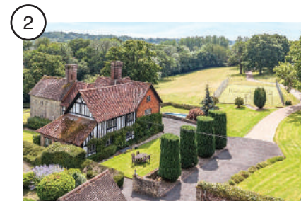
Area 2 - Resurface tarmac
