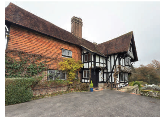
C17th range (western wing & southern gable)
