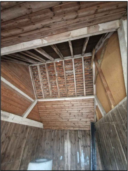
Interior photo of existing timberboard finish (portion) in former annexe (area 1b)
