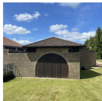
The eastern end of the Narthex is infilled with timber and faces in the direction of the car park
