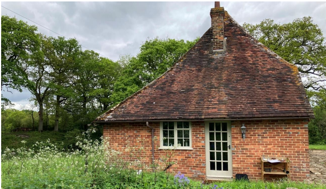
Figure 5 – Existing south elevation
