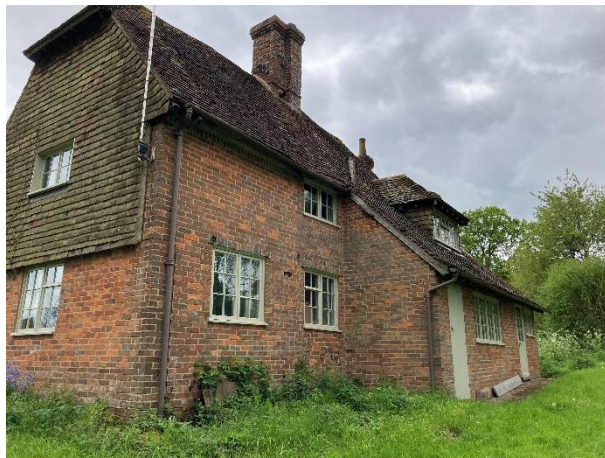
Figure 8 – Existing northwest corner
