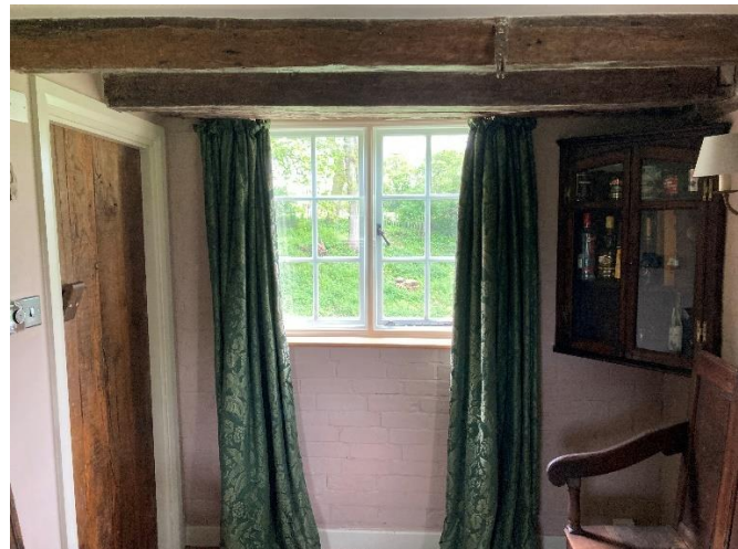
Figure 18 – Existing window and external wall to be removed to provide access into new extension
