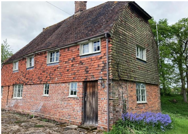
Figure 2 – Existing northeast corner
