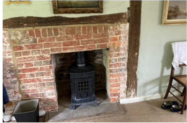
Figure 7 – Existing first floor fireplace
