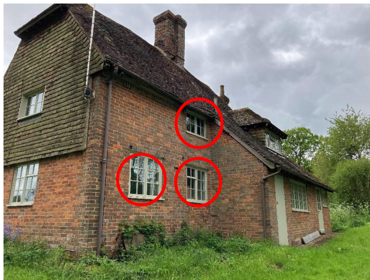
Figure 13 – Existing ground and first floor windows to be removed to enable proposed extension.
