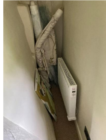
Figure 24 – Existing recess next to chimney stack
