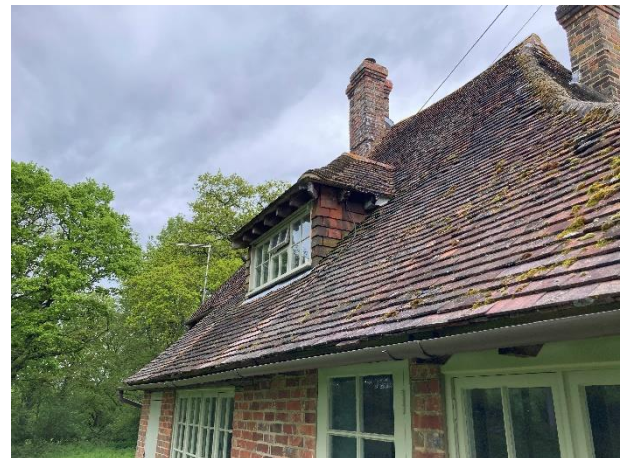
Figure 9 – Existing dormer window
