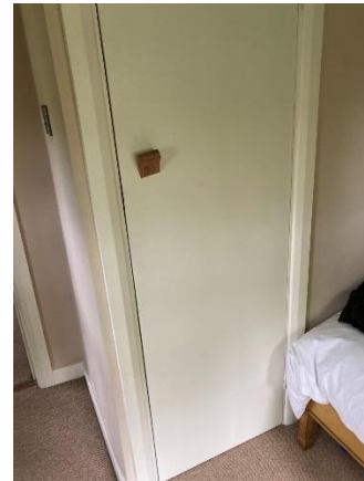
Figure 21 – Existing cupboard and internal wall to be removed
