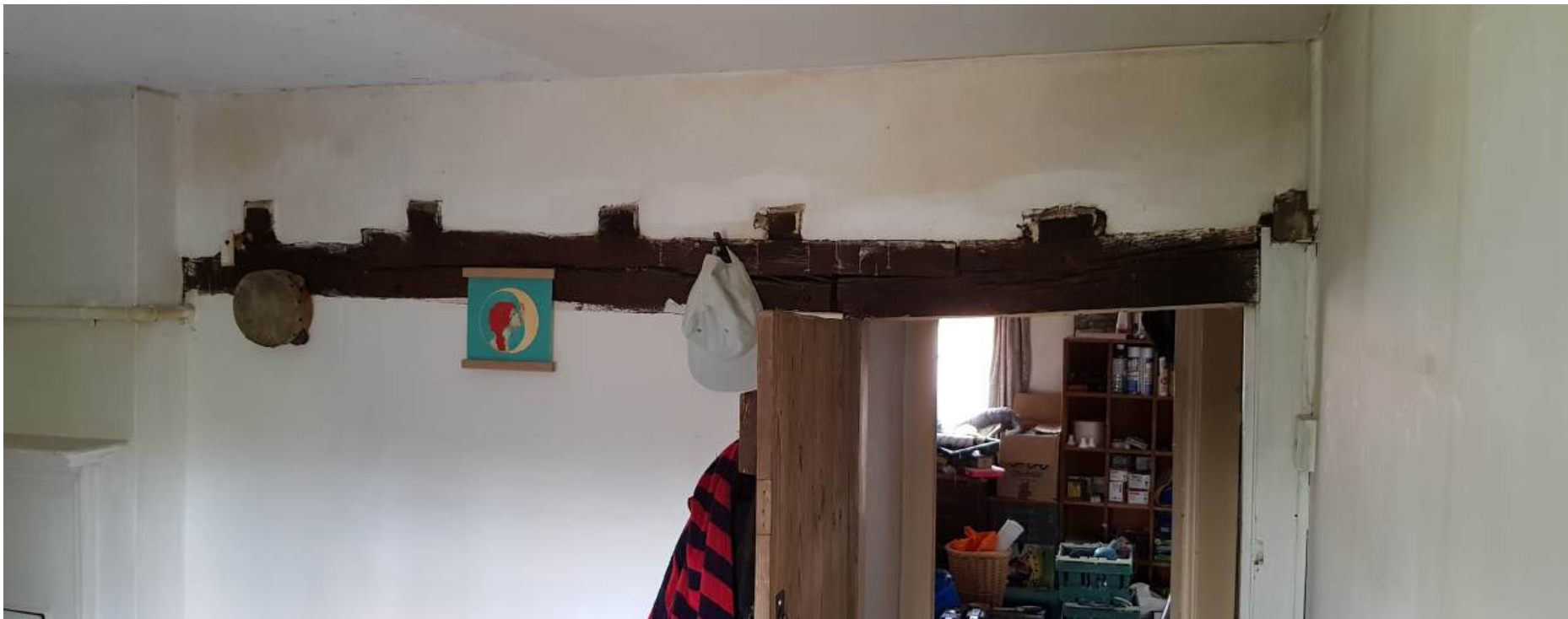
REAR BEDROOM (FORMER WALL PLATE)
