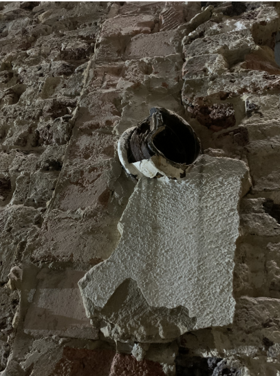
Example of SVP connection cut SVP 3 second floor area where historic bathroom was located
