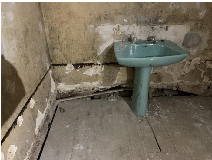
Examples of 70s plumbing additions including supplies and drainage tracking around rooms and penetrations through fabric.
