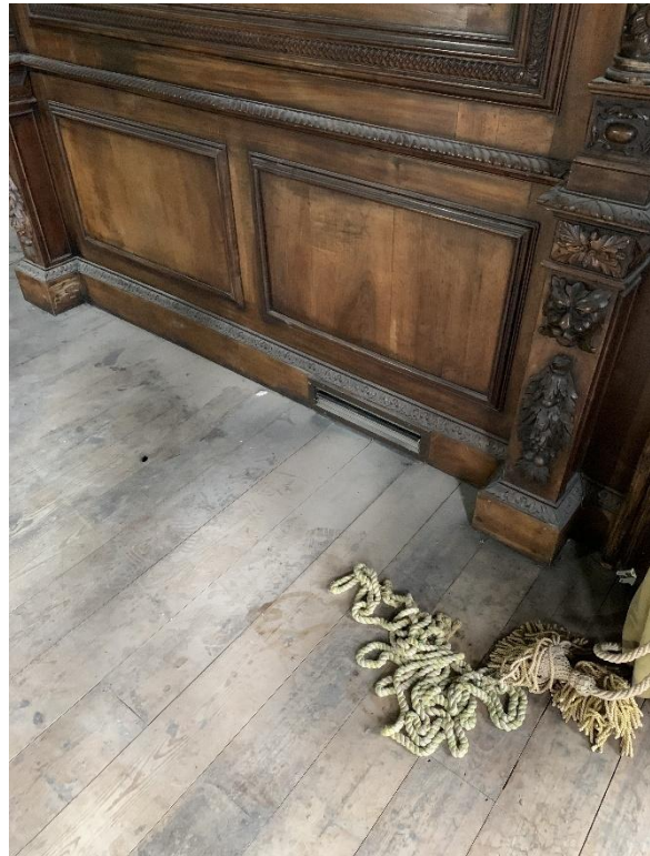
Non-original grille, connected to the duct system
