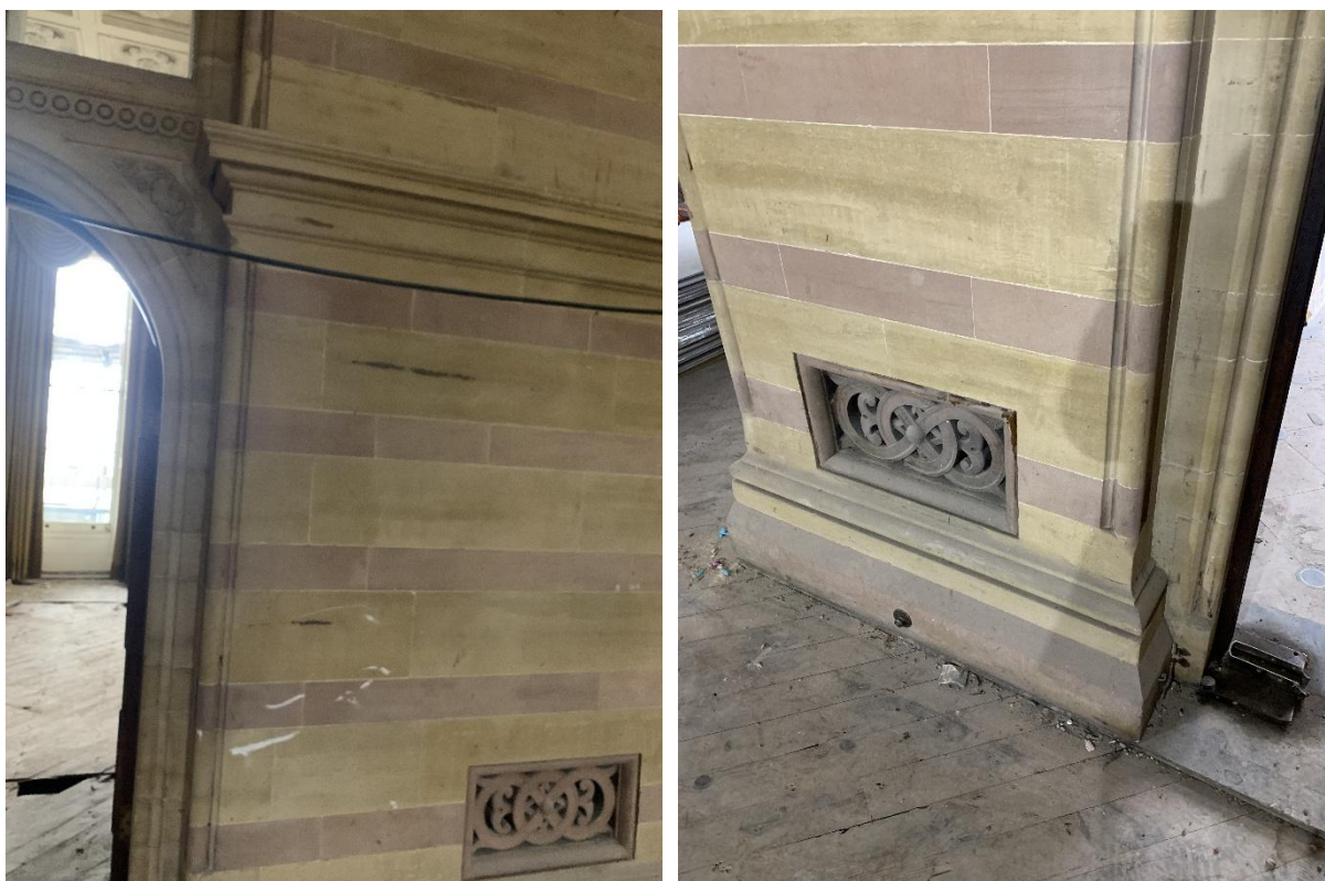
Retained existing stone grilles in the entrance hallway
