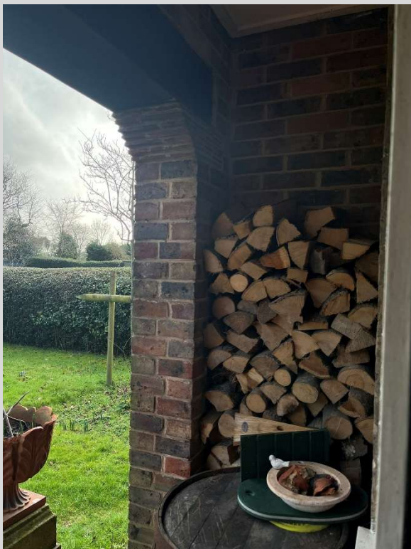
30 January 2026, 13:25 — SE door recessed 93cm under covered entrance
