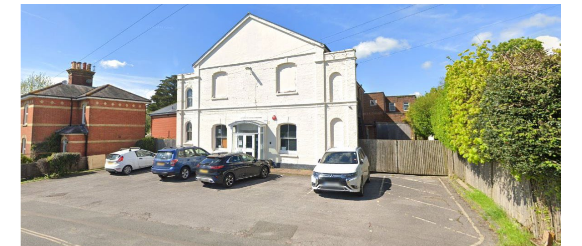
Picture of the existing
