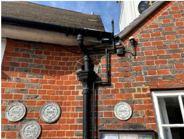
External rainwater goods (gutters and downpipes) tend to be black.
