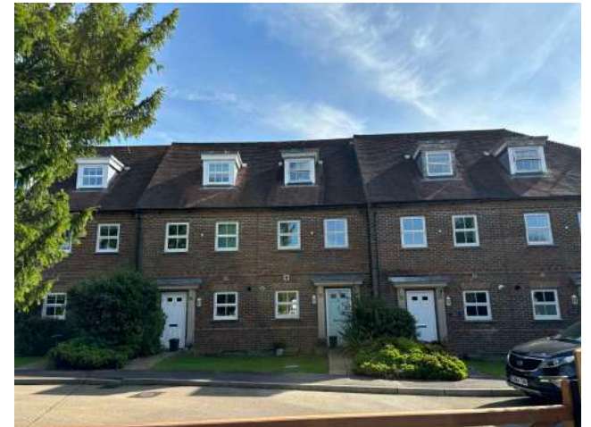
Flat roof dormers providing both natural light and additional headroom to rooms in the roof.
