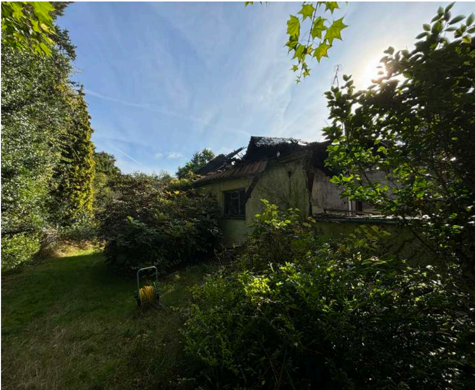
Northwest corner of building.
