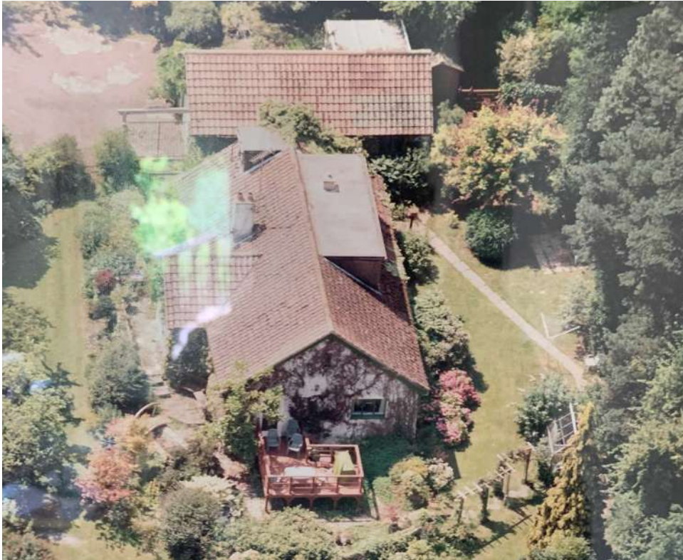
Aerial photograph of dwelling prior to fire
