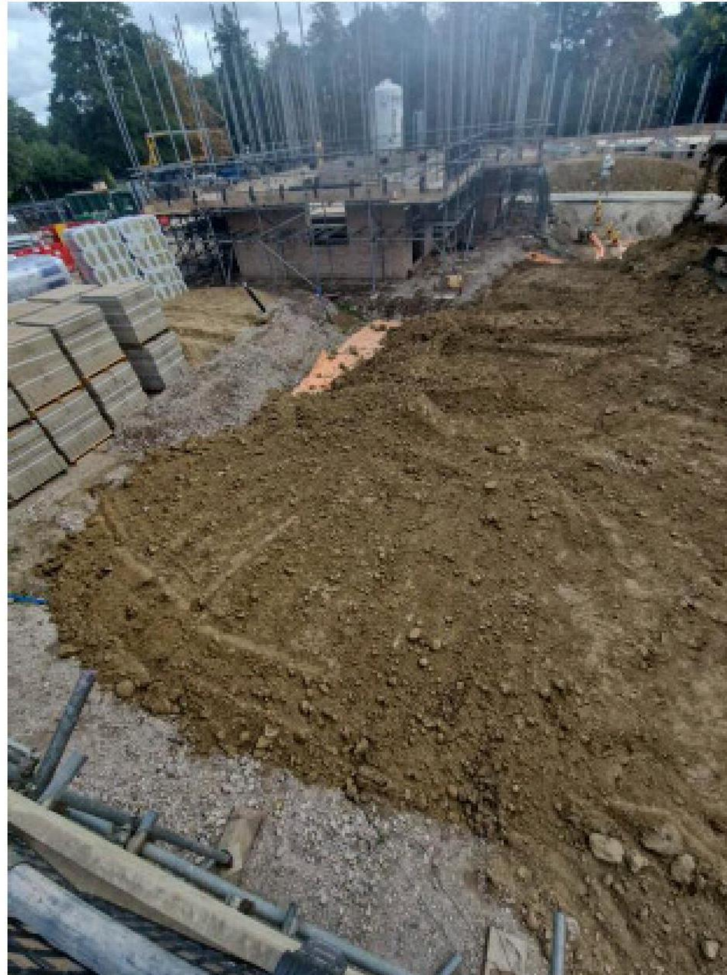
Photograph 3: Placement of clean materials over geotextile within Plots 7 and 8.
