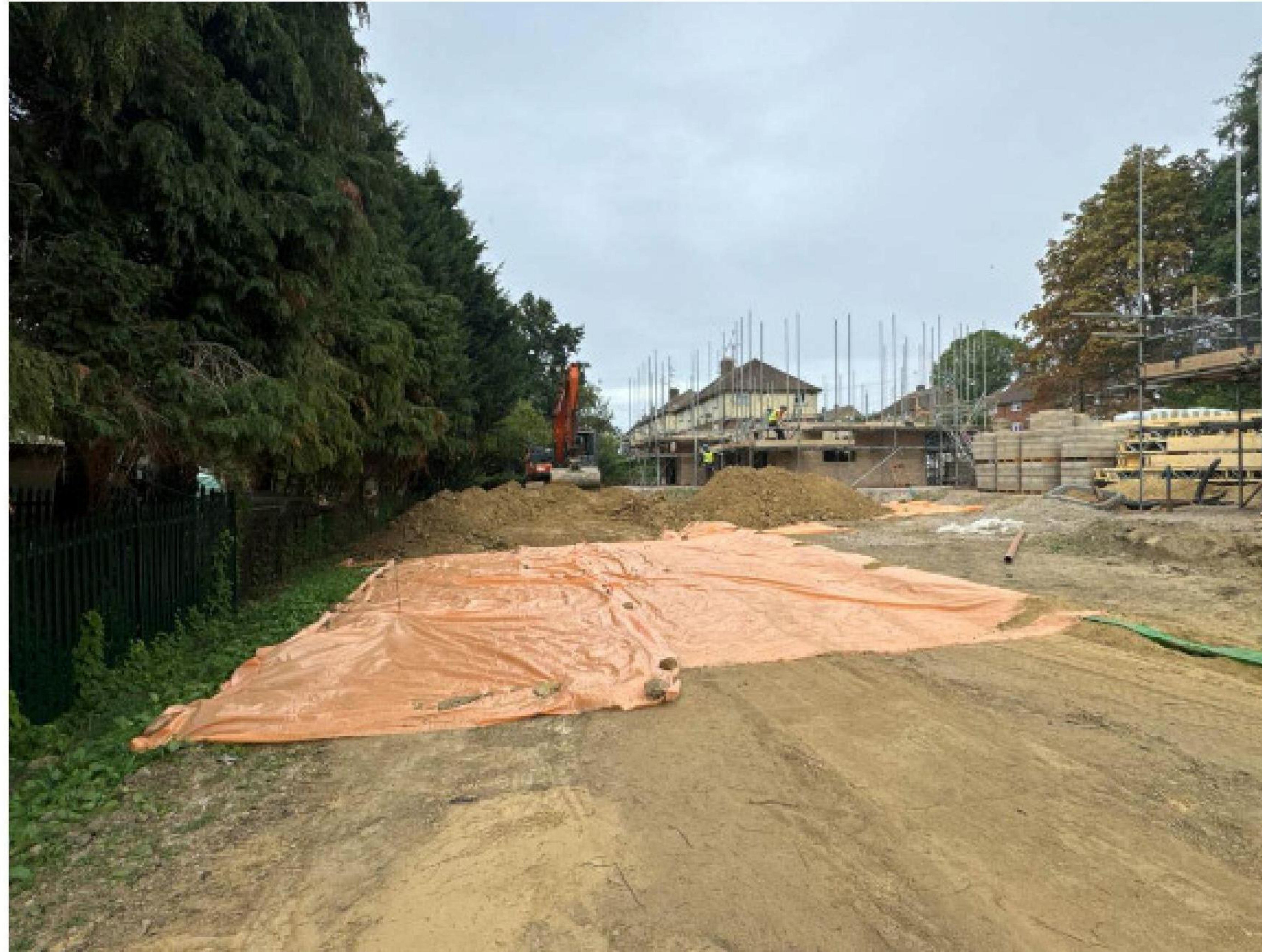
Photograph 1: Placement of geotextile within Plots 8, 9 and 10.
