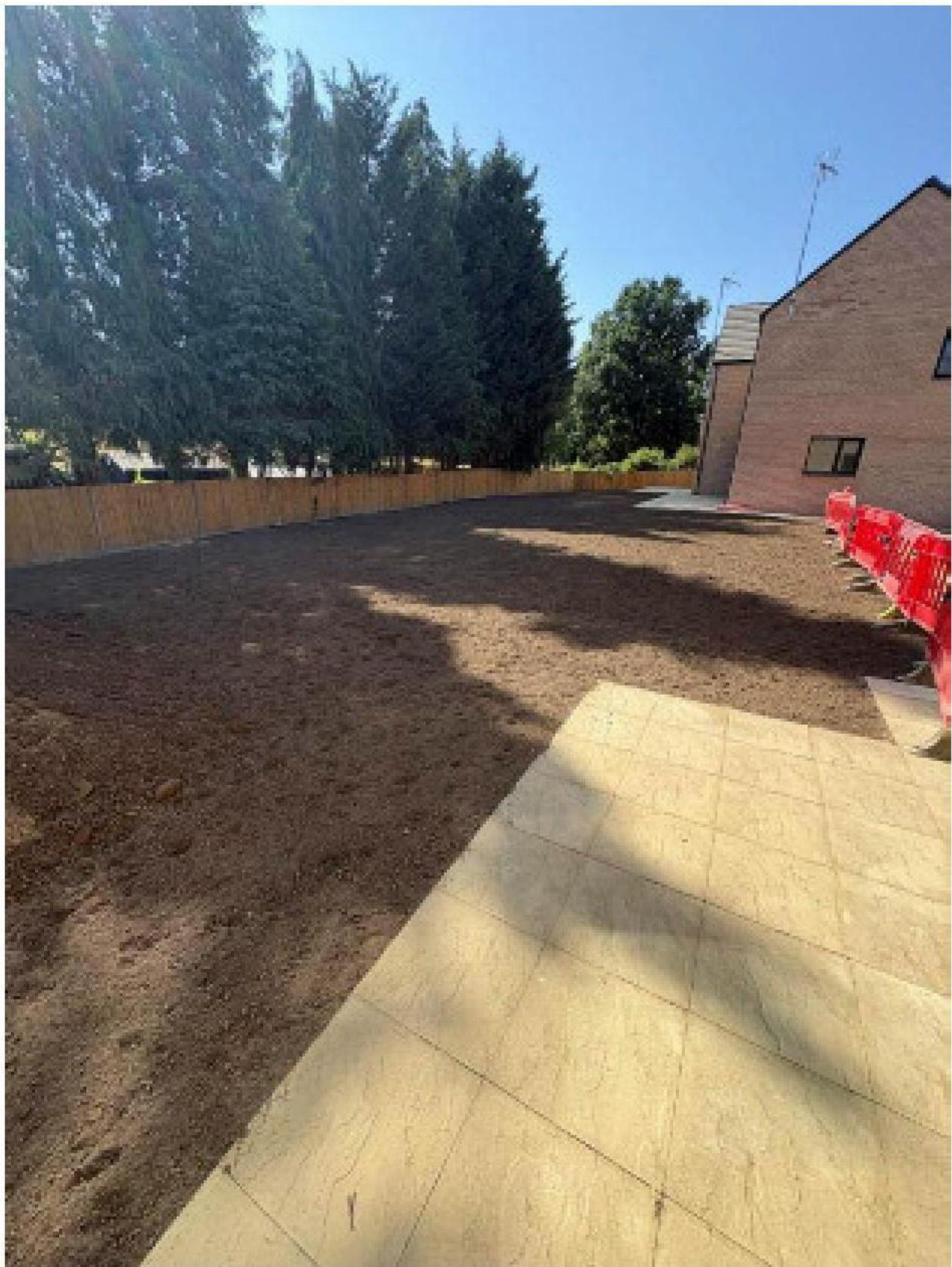
Photograph 7: View of finished soft landscaping and hardstanding associated with rear gardens of Plots 7-10 prior to seeding.
