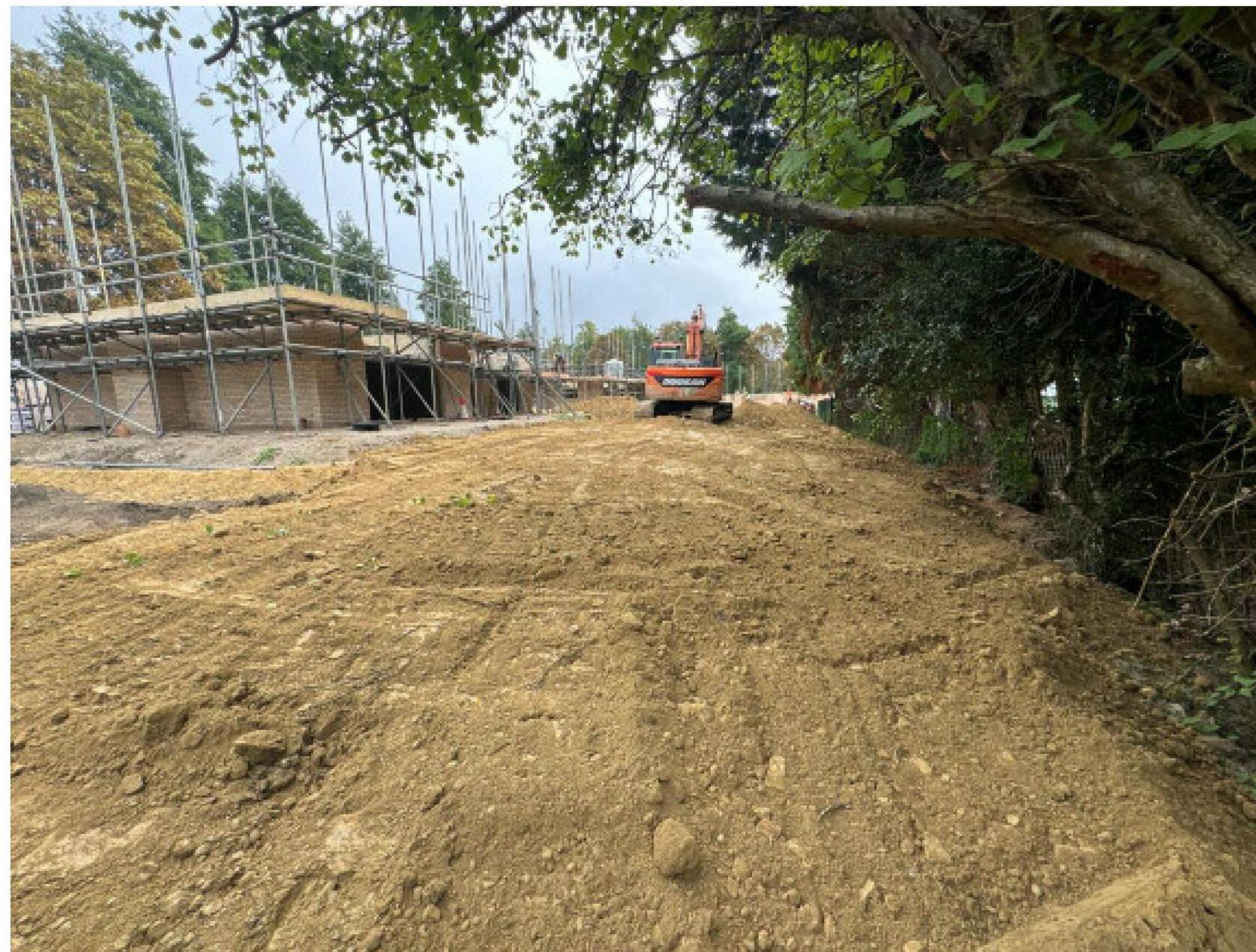
Photograph 4: Placed materials within Plots 7 and 8 over geotextile.
