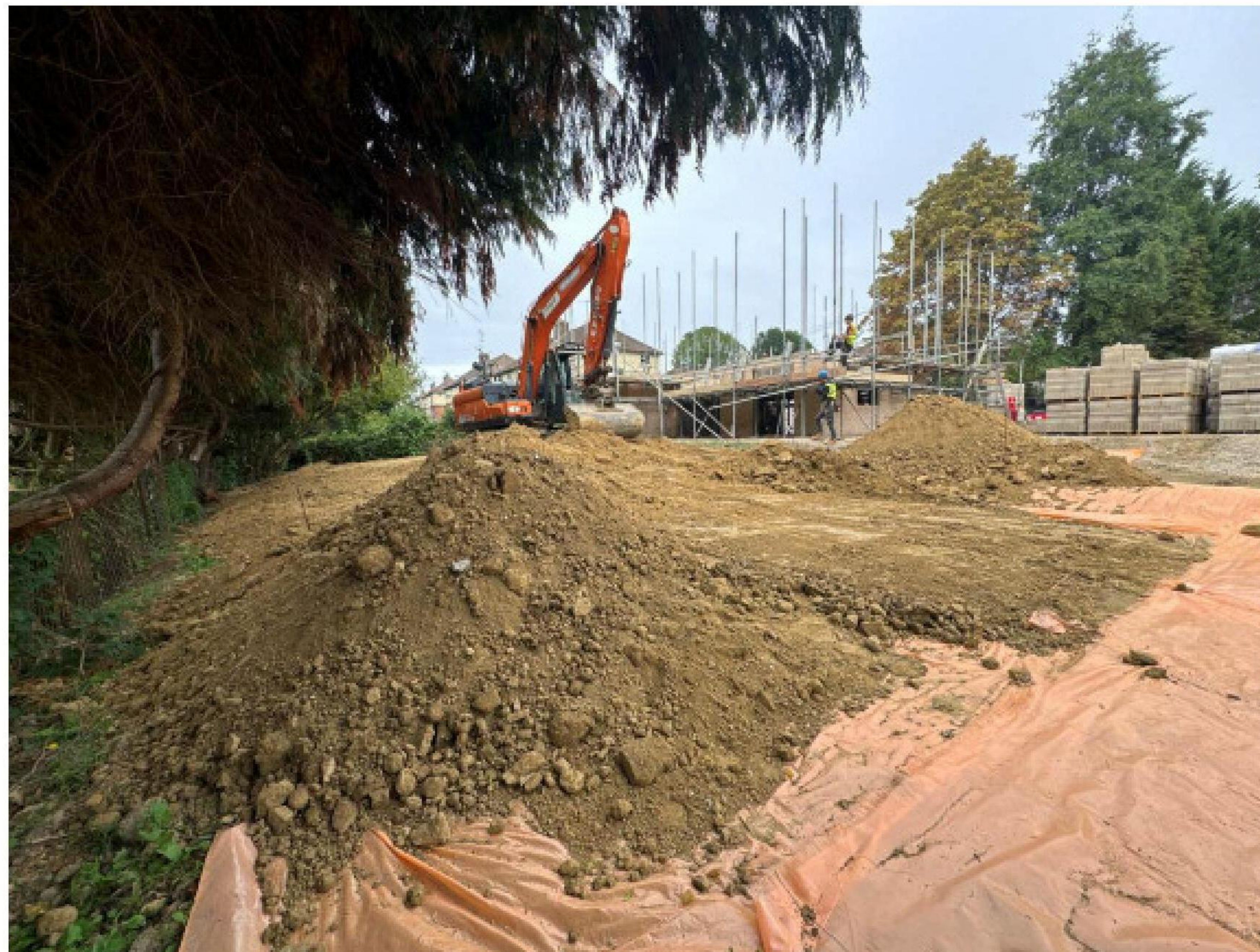
Photograph 2: Placement of clean materials over geotextile within Plots 9 and 10.
