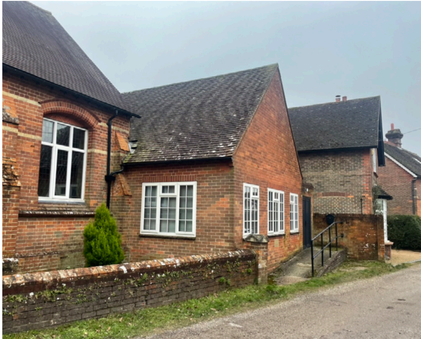
Existing gable end
