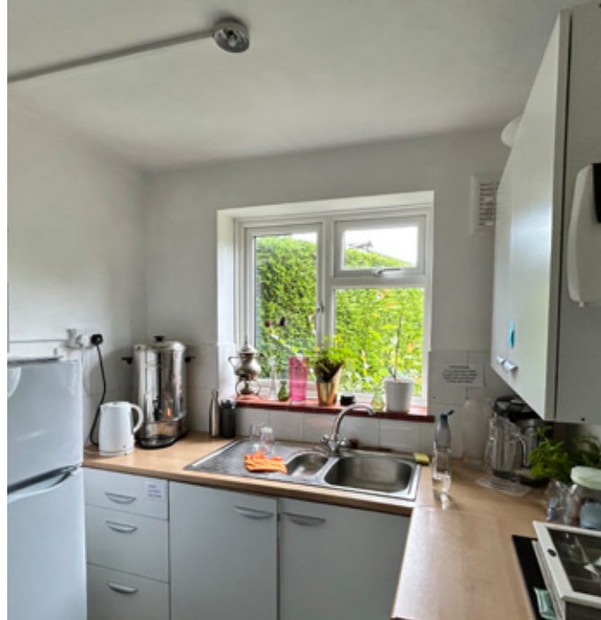
4. Existing kitchen area with view towards rear garden
