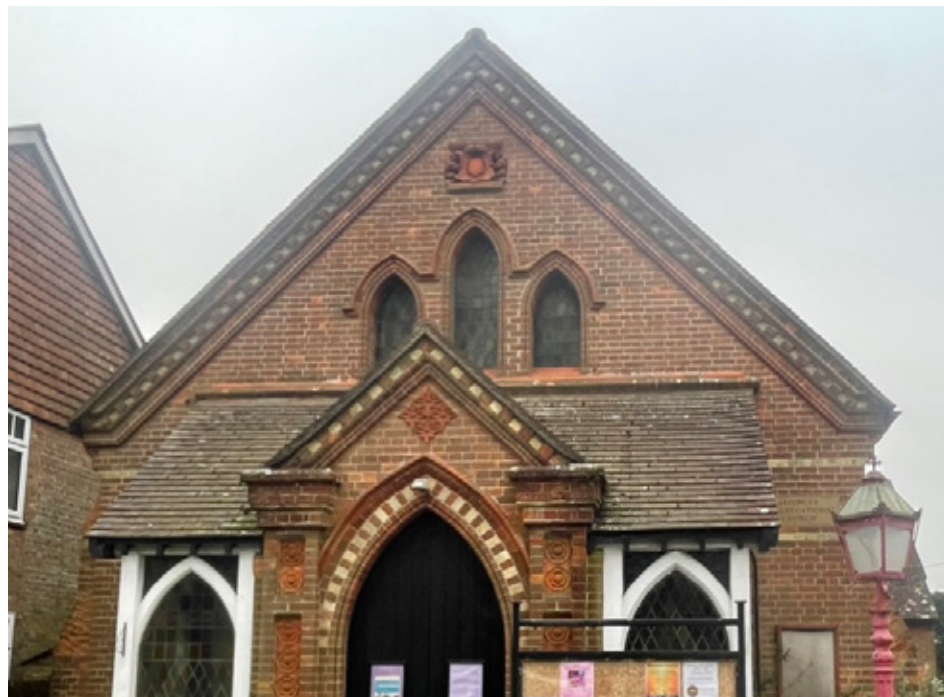
4. View ornate detailing present on existing building facade
