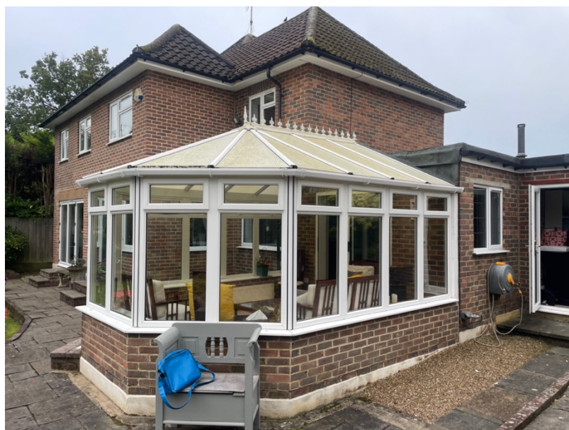
3.1 - Image showing the conservatory and rear of the garage.
