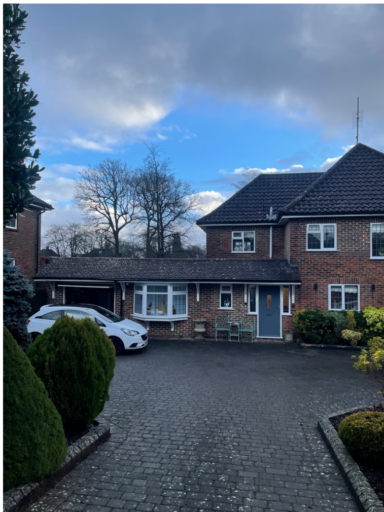
3.2 - Image showing the front of the property including the garage on the left.
