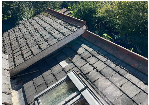
Existing Roof Tiles
