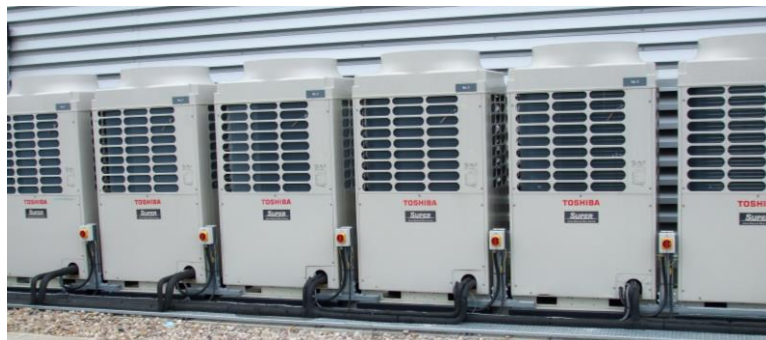
Figure 13: Example of ASHP condenser units
