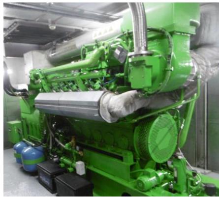
Figure 11: Example of a CHP engine
