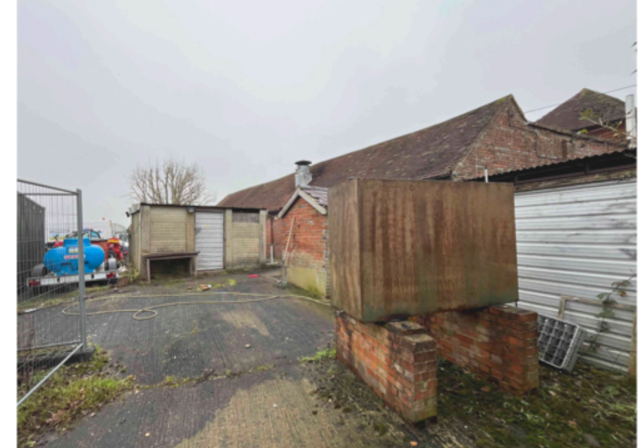
West Elevation viewed from the south
