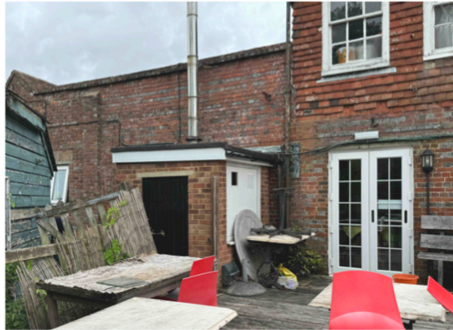
South Elevation (Stables and farmhouse junction)
