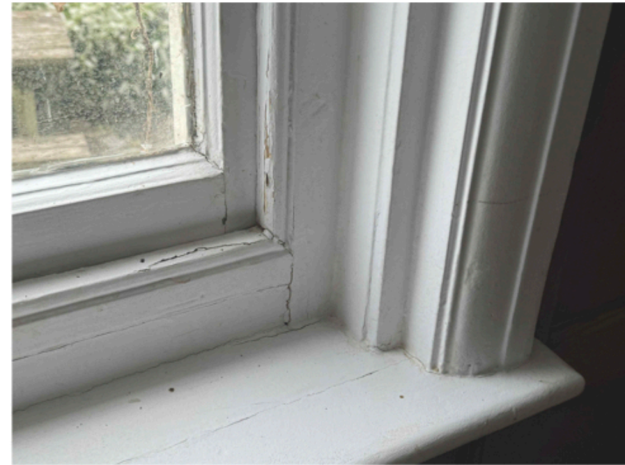
Typical sash window
