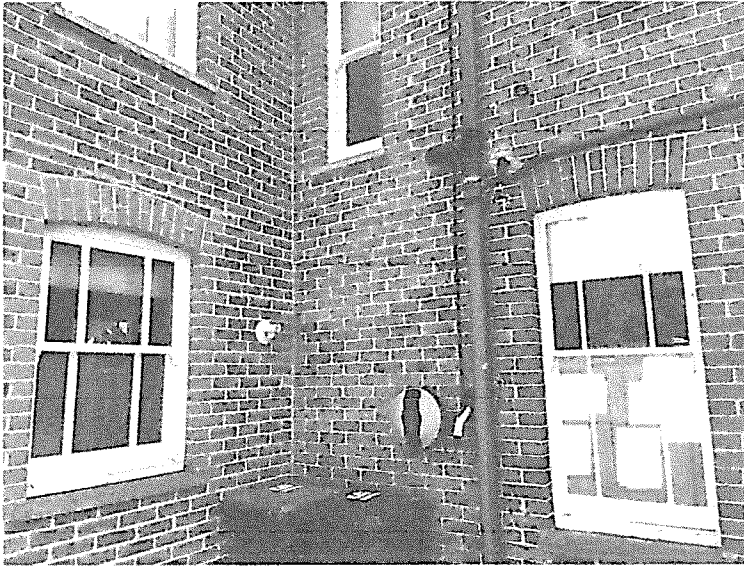
EXTERIOR SHOWING ORIGINAL 1907 AND 2009 WINDOW VERSIONS TOGETHER
