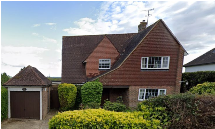
Hanging tiles facade with mixed brick along Fox Hill Close
