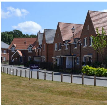
Well overlooked by adjacent houses
