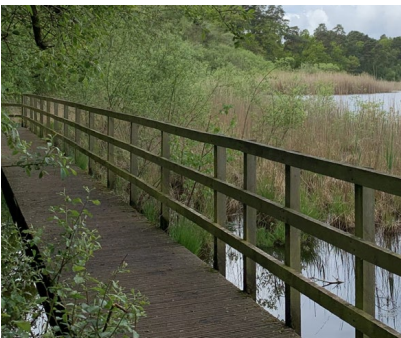
Boardwalks across existing water feature, fenced and gated.
