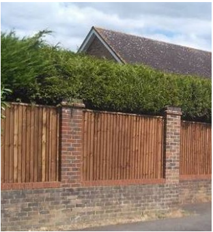
Brick wall with timber panel
