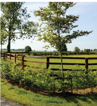
Timber post and rail to restricted access areas
