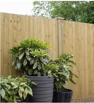
Close-board timber fence
