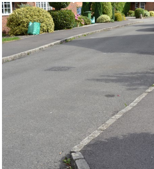
Bitmac to primary roads and pavements
