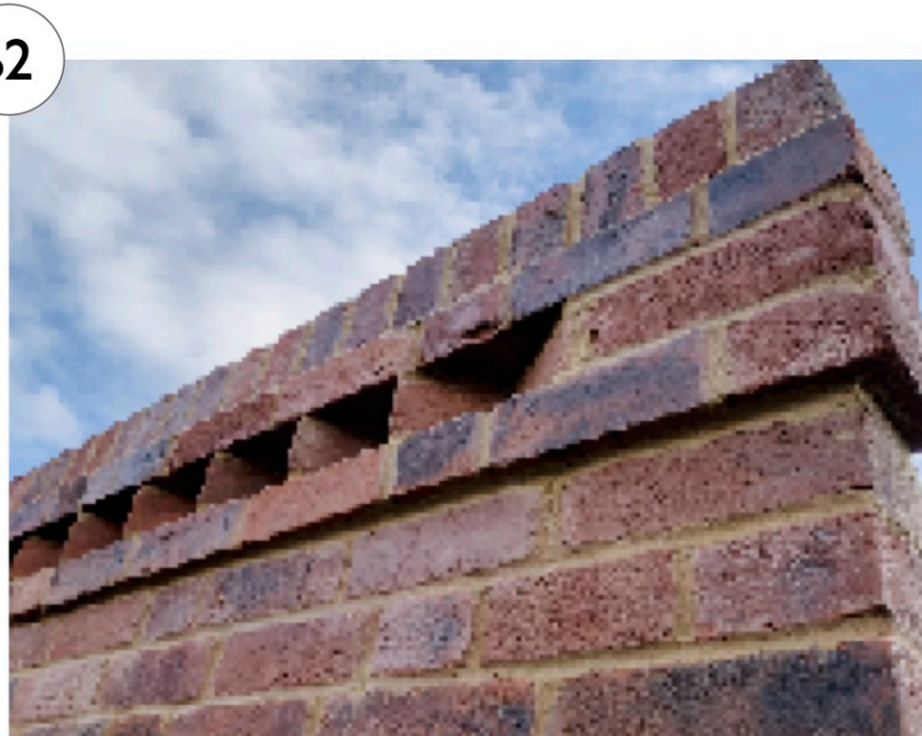
1.2M BRICK BOUNDARY WALL
