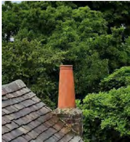
Original bake house chimney
