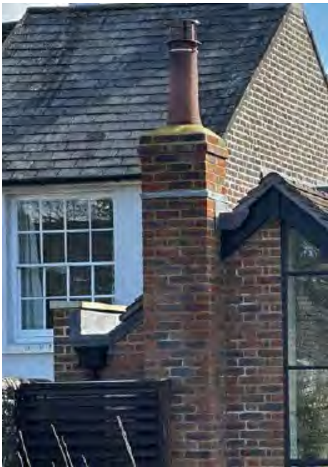
Recent photograph of parapet wall detail
