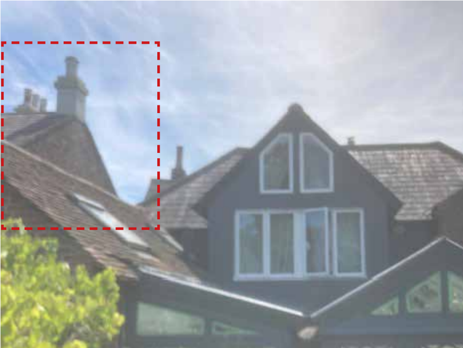
109 High Street south gable wall before re-pointing
