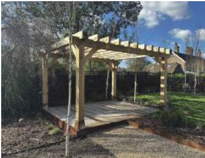
Recent photographs of the timber pergola
