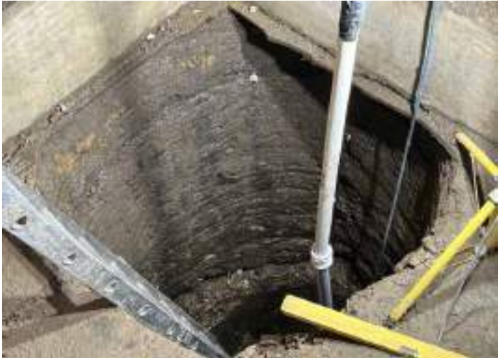
Opened well shaft
