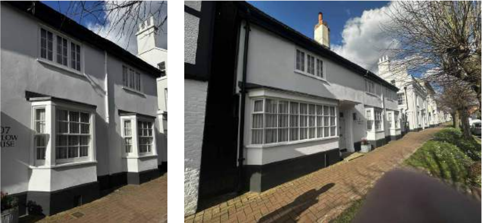
Photographs of front elevation after restoration works
